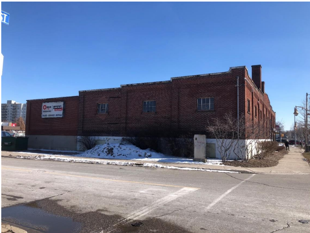
Figure 4: A view of Schnurr Electric from northwest, taken from corner of Gordon and Surrey Street. White stucco is visible on the foundation.
