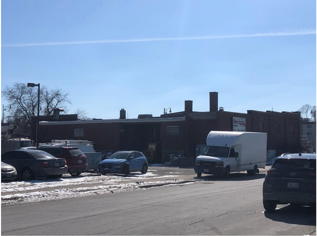
Figure 5: View of loading bay and stockyard for Schnurr Electric, taken from opposite side of Surrey Street to the northeast. Several cars, vans, and delivery vehicles are visible in this image.
