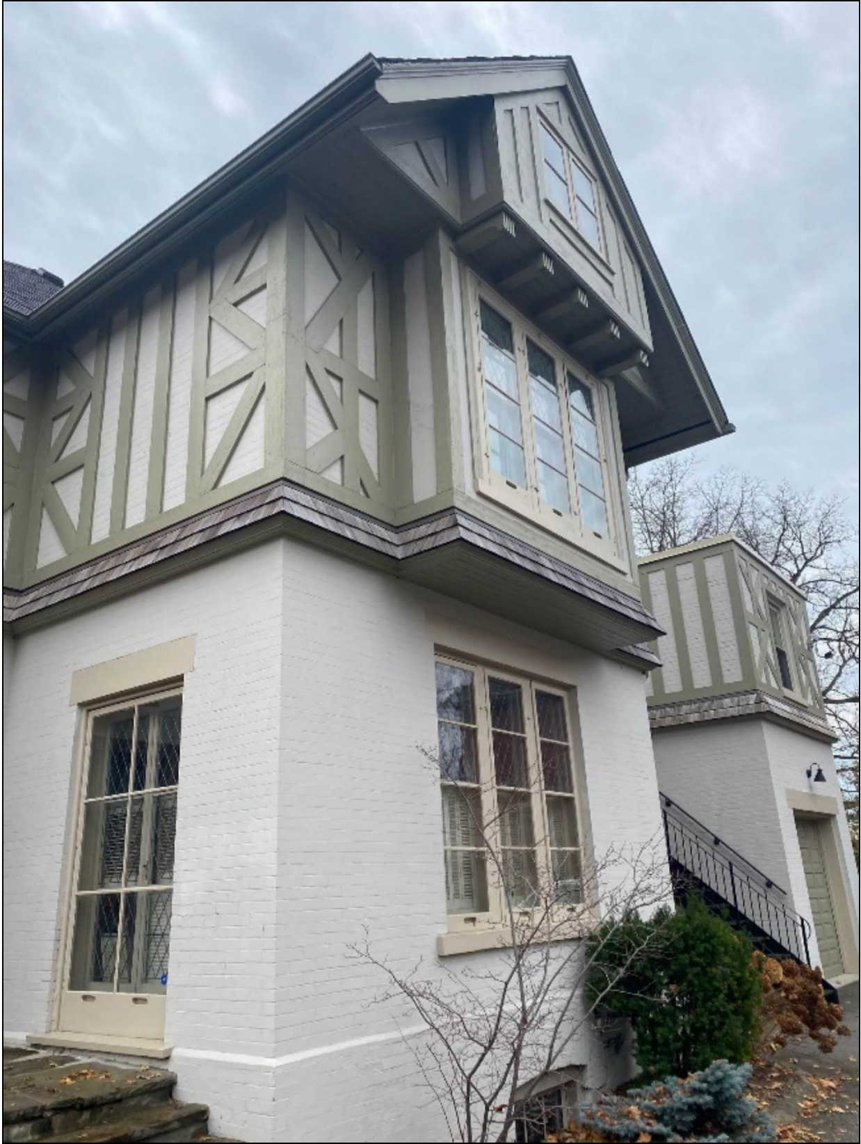
Figure 2: North facing protruding bay at 100 Queen St (photograph: Heritage Staff, 2024)
