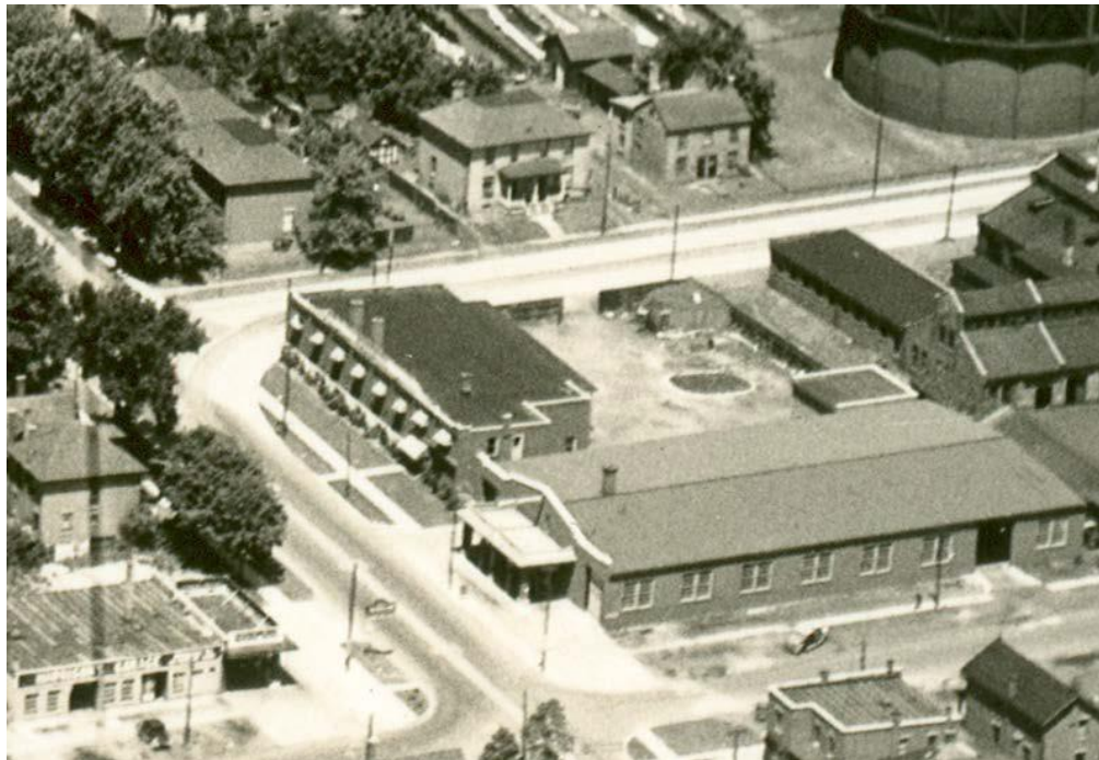
Figure 25 Detail from an aerial photo from 1931. Visible is MacKey's Bakery (by this time occupied by Dominion Bakeries). To the south is Brown's Transport and other nearby industrial buildings, now all lost. Photo: City of Guelph.
