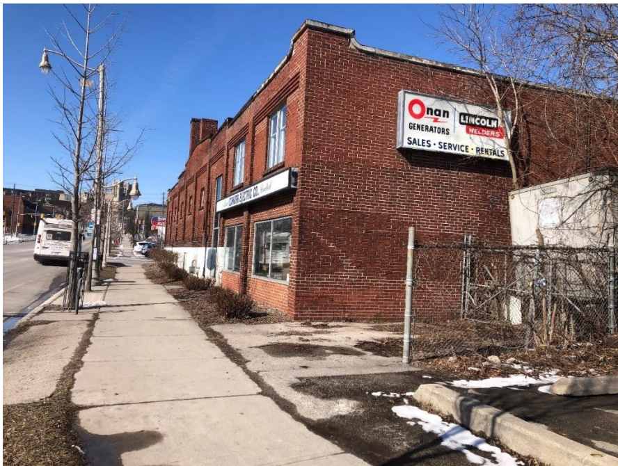
Figure 2 View of Schnurr Electric from southwestern corner. Several visible signs, with the end of a tractor trailer visible on right side of image.
