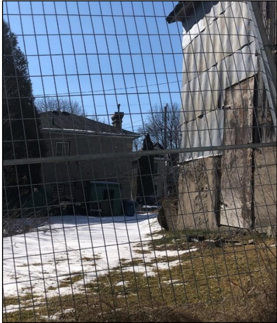
Figure 14: View of 14 Neeve Street barn and stone house through a construction fence. Cedar trees on left of photo, a small green veranda covers rear entrance to stone house.
