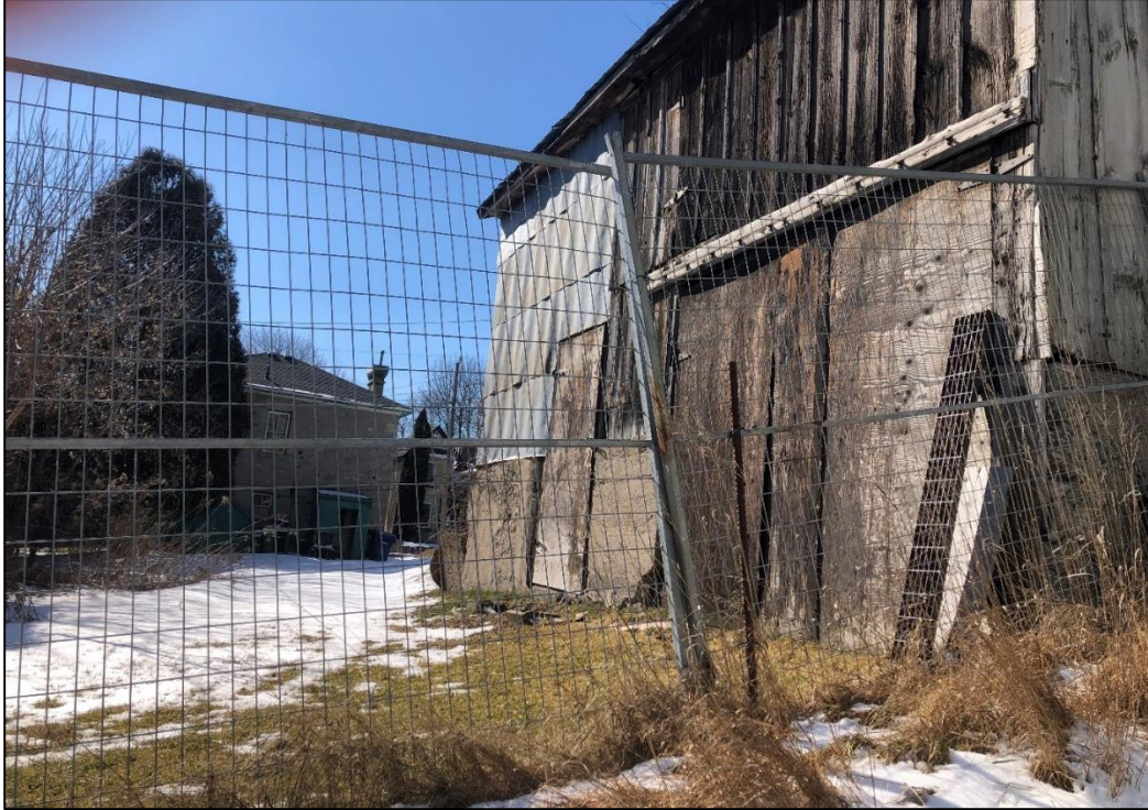
Figure 13 View of 14 Neeve Street barn and rear of stone house
