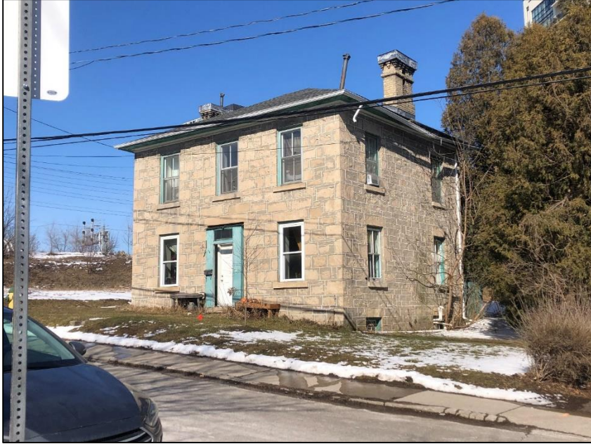
Figure 7: Photo of 14 Neeve Street Neeve Street.
