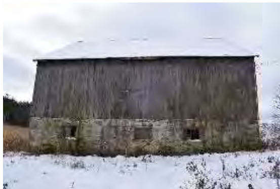
Plate 81: East elevation looking west
