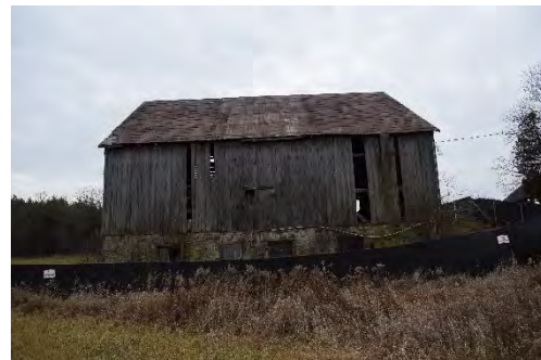
Photo 4-10: East elevation looking west
