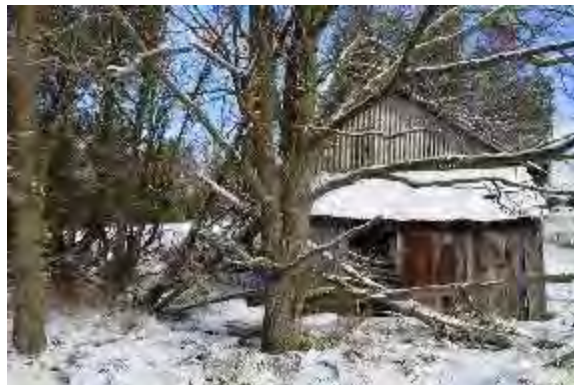
Plate 149: Outbuilding looking east
