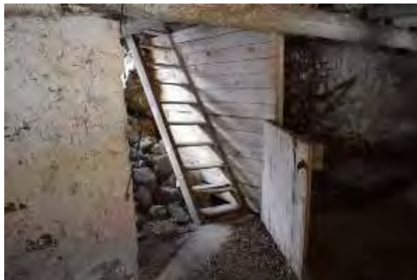
Plate 127: Wood staircase to lower storey in stone tail
