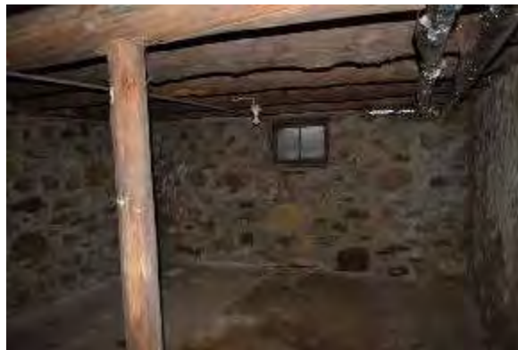
Plate 54: Basement looking east
