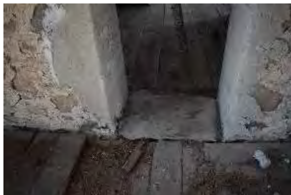
Plate 114: Stone threshold between timber frame barn and stone tail
