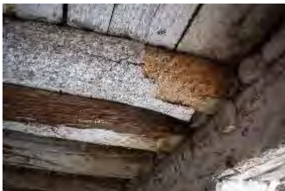
Plate 144: Old growth beams supporting upper threshing floor
