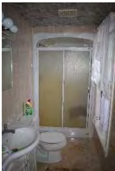
Plate 63: Second storey bathroom looking south
