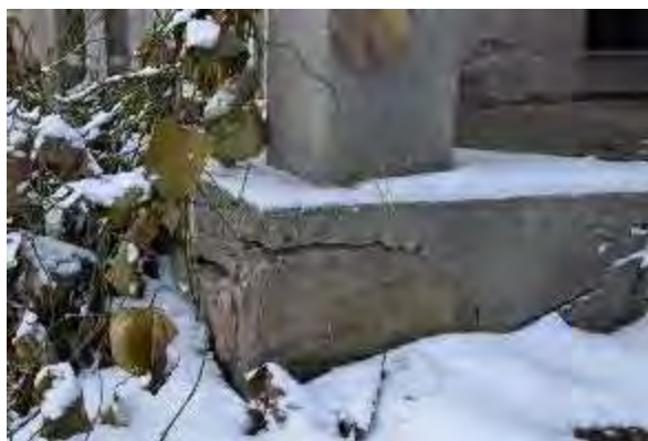
Plate 33: Stone porch base
