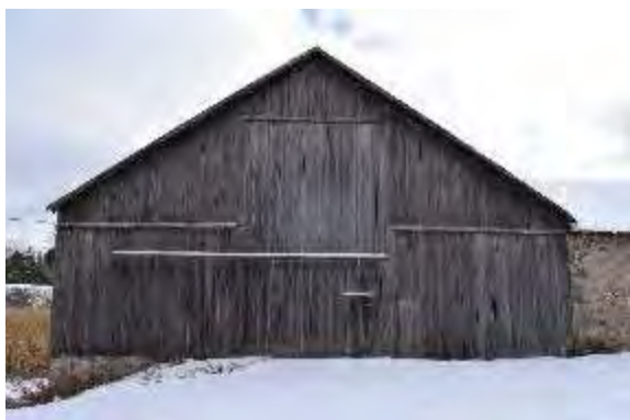
Plate 72: North elevation looking south
