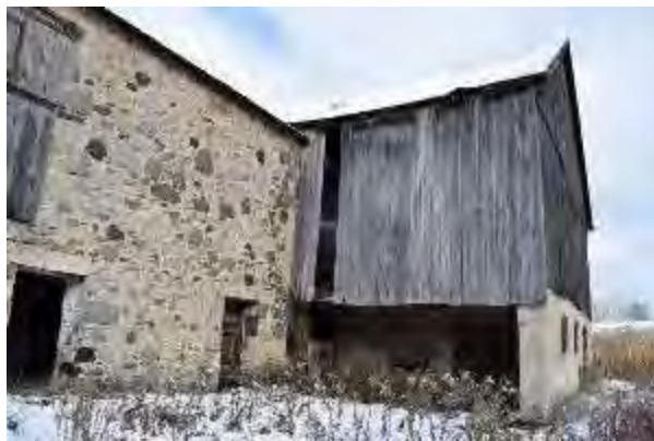
Plate 87: Southwest corner of timber frame portion of barn looking east
