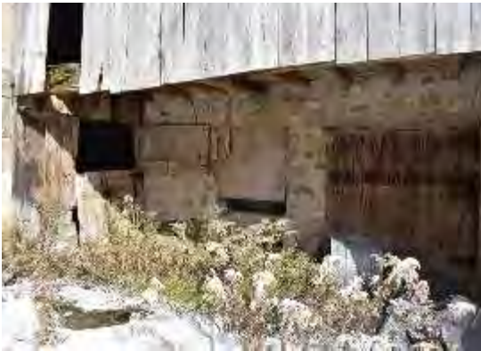
Plate 88: Southwest corner of timber frame portion of barn looking east
