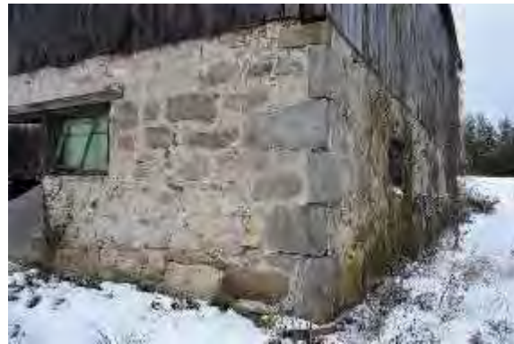
Plate 71: Close-up of stone foundation
