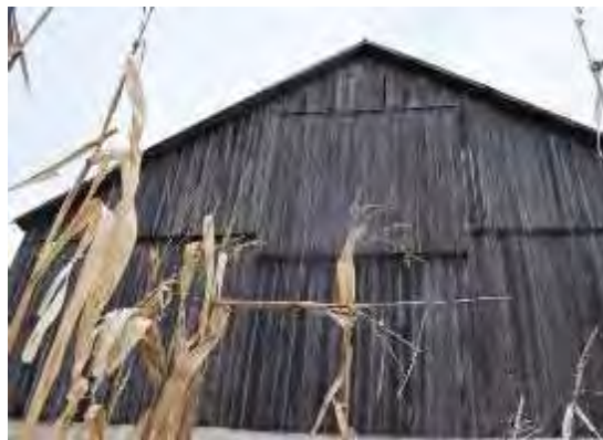
Plate 86: South elevation of barn looking north
