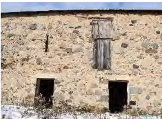
Plate 90: South elevation of stone tail looking north
