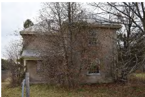
Photo 4-1: Front (east) elevation looking west
