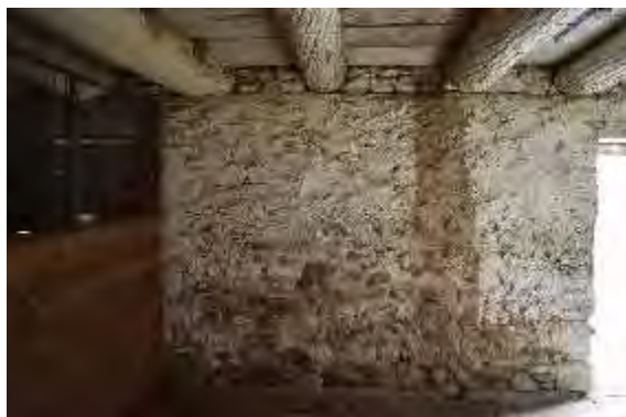
Plate 145: Old growth beams supported by stone wall looking south
