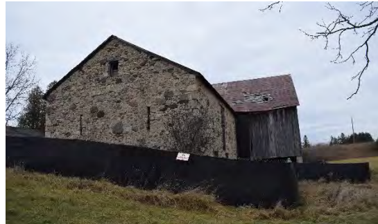
Photo 4-8: West elevation looking east
