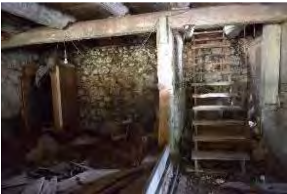
Plate 126: Wood staircase from timber frame portion of barn to lower stables
