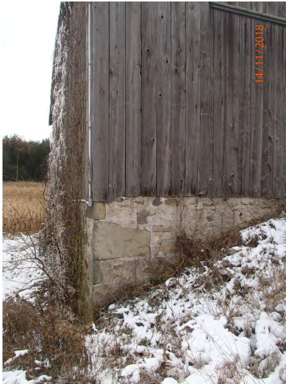
Photograph No. 20 – Northeast corner, fair condition
