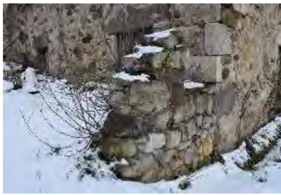
Plate 95: Stone wall on southwest corner
