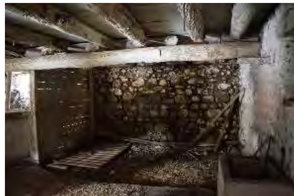
Plate 139: Lower storey of stone looking north
