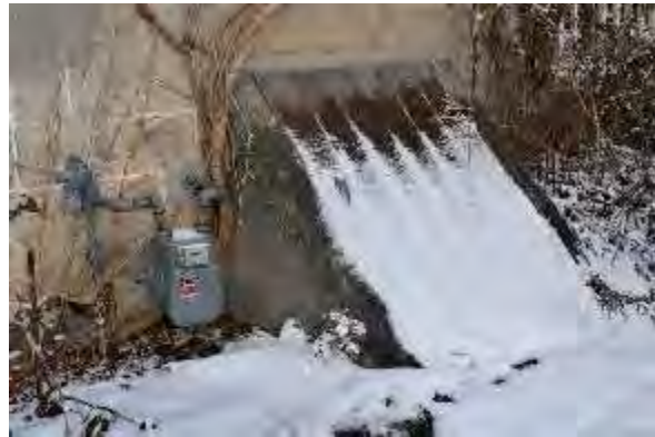
Plate 40: Exterior basement hatch
