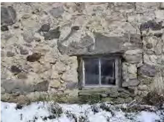
Plate 94: Window on west elevation
