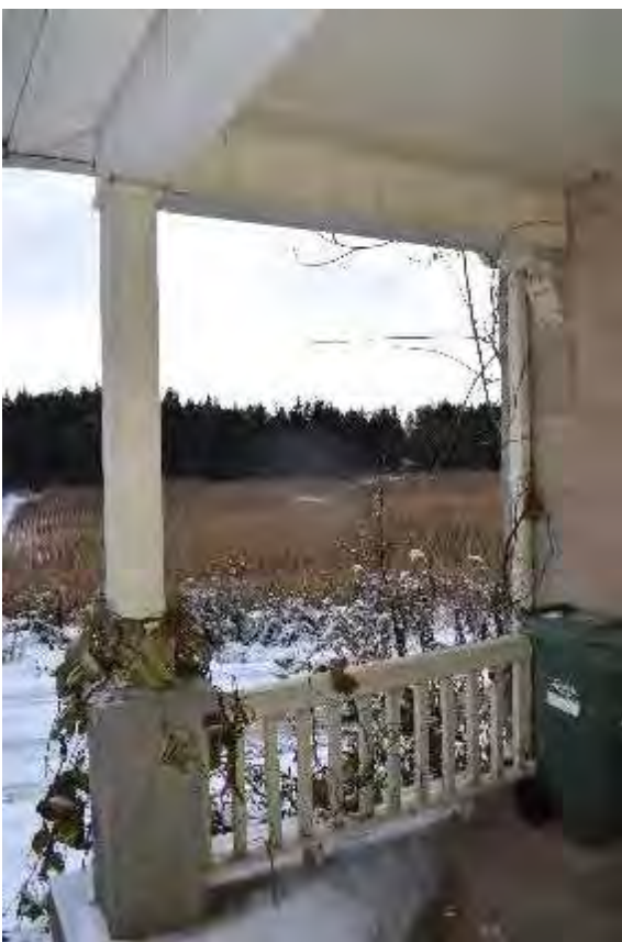
Plate 32: Front porch pier, column and railing looking southwest
