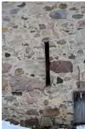
Plate 77: Close-up of slit window
