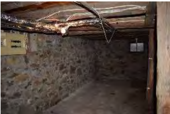
Plate 53: Basement looking east
