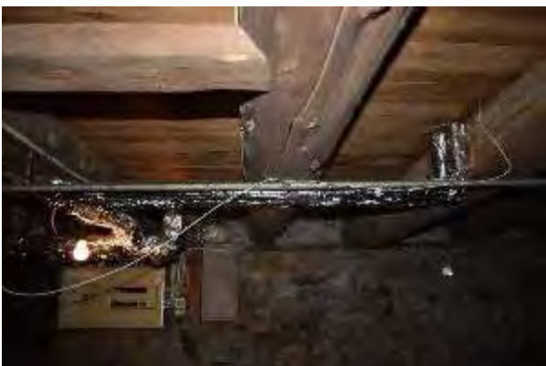
Plate 55: Wood beams looking north
