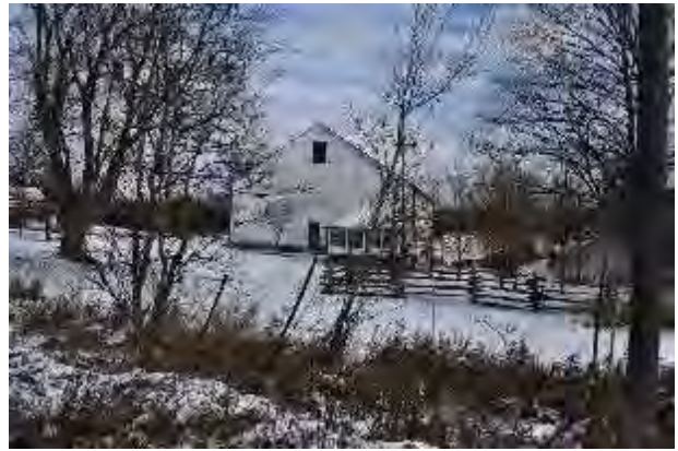
Plate 7: 2162 Gordon Street barn looking northeast
