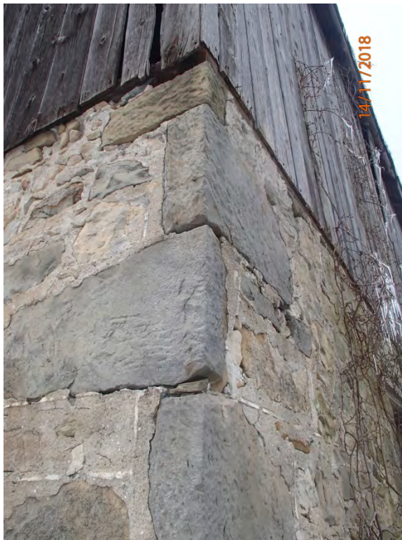
Photograph No. 21 – Southeast corner, fair condition
