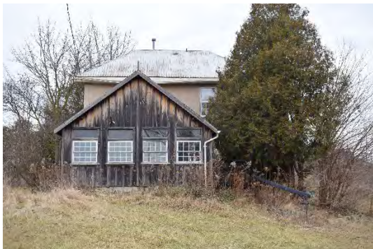
Photo 4-3: West elevation looking east
