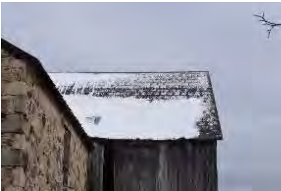
Plate 70: Close-up of tin cladding on roof
