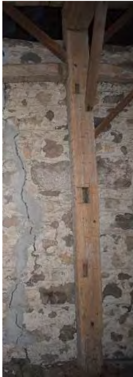
Plate 101: Hand hewn beam and joints
