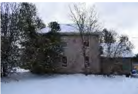
Plate 35: North elevation looking south
