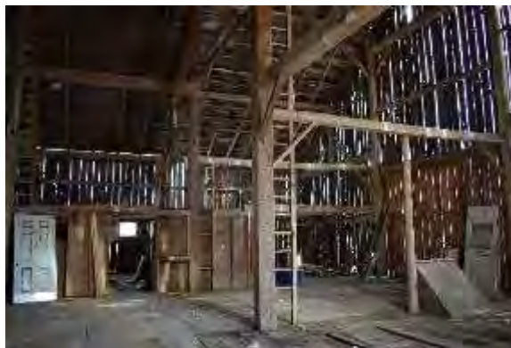
Plate 97: Threshing floor of barn looking southeast
