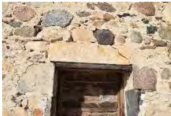
Plate 91: Close-up of stone lintel above door
