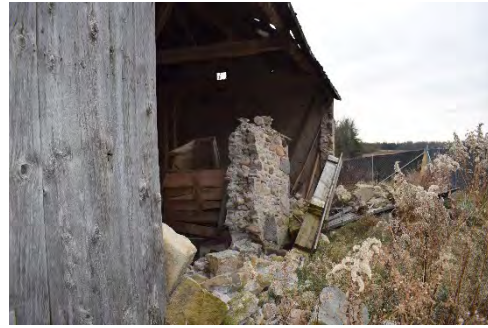
Photo 4-6: North elevation looking southwest
