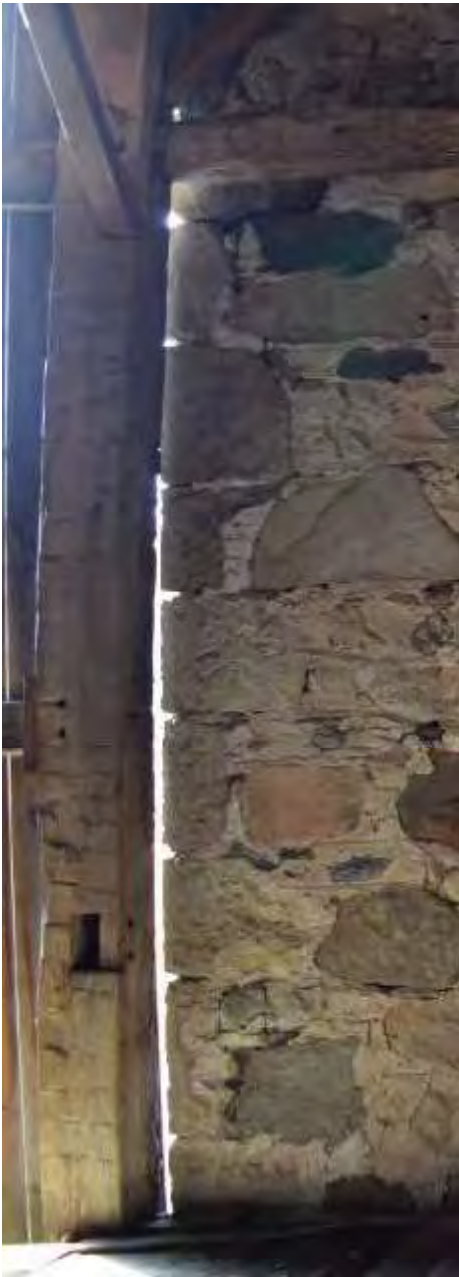
Plate 100: Hand hewn beam and joints
