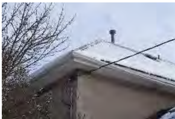
Plate 25: Metal chimney and wide eaves from northwest corner
