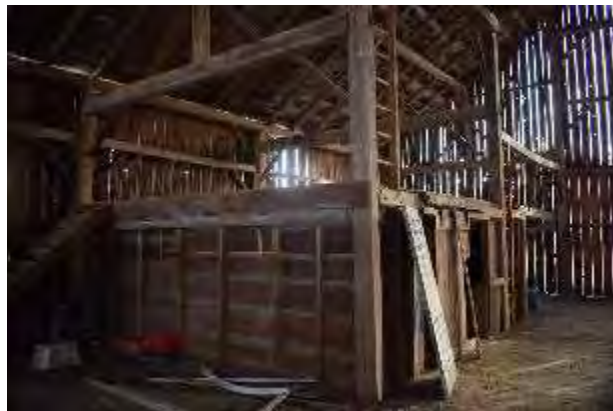
Plate 103: Grain storage area looking southeast
