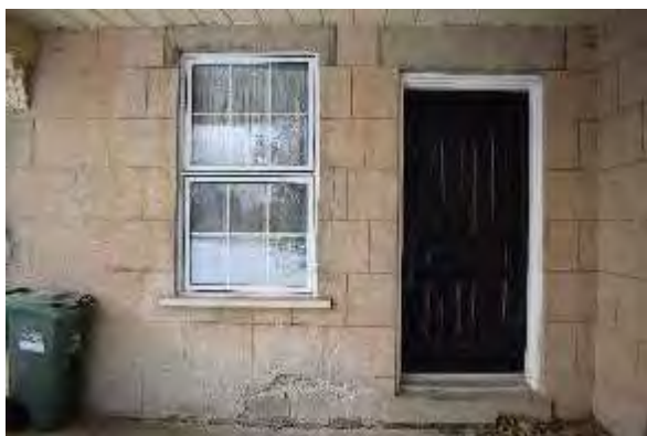
Plate 28: Front door and with concrete lintels and sills
