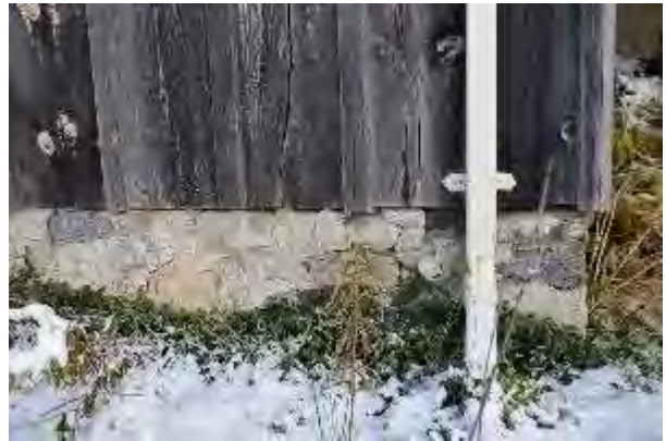
Plate 38: Close-up of addition foundation
