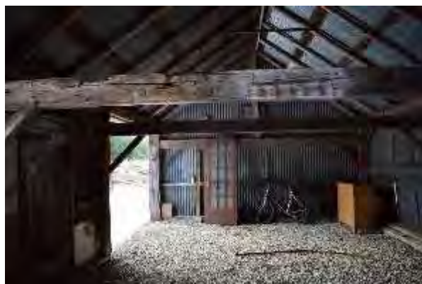
Plate 153: Outbuilding interior looking west
