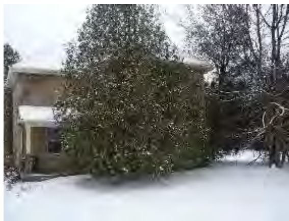
Plate 9: Front (east) elevation of residence looking west
