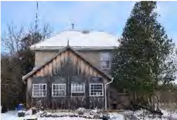
Plate 37: West elevation looking east
