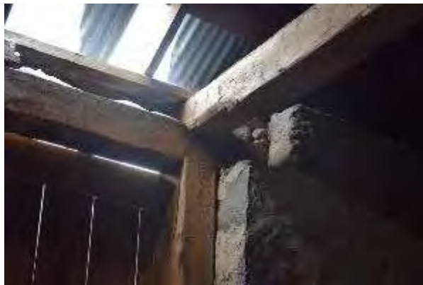
Plate 121: Stone tail beam on door frame
