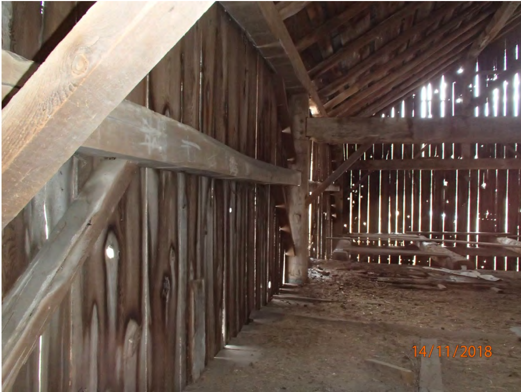
Photograph No. 12– Mezzanine and West wall framing (fair condition)
