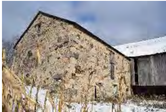
Plate 89: Southwest elevation looking northeast
