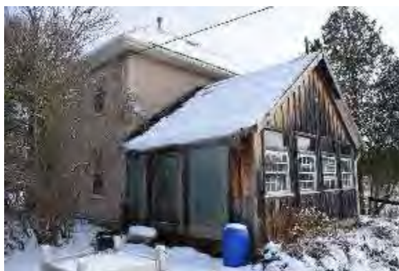
Plate 36: Northwest elevation looking southeast
