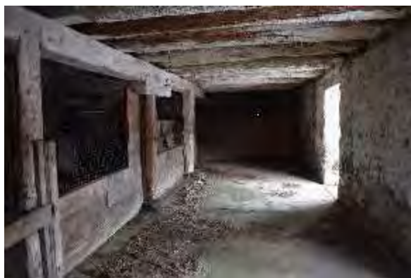
Plate 141: Lower stables in stone tail looking east
