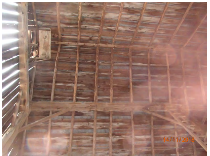
Photograph No. 13 – Superstructure barn roof framing (fair condition)
