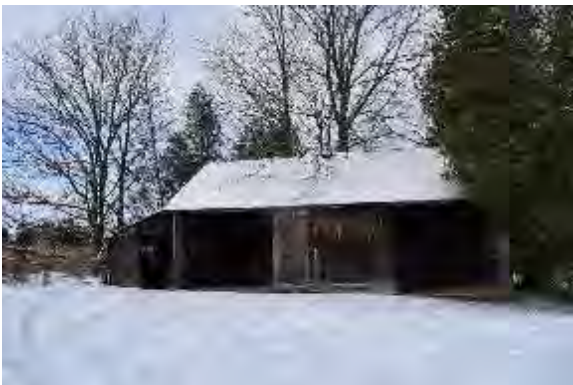
Plate 148: Outbuilding looking northwest
