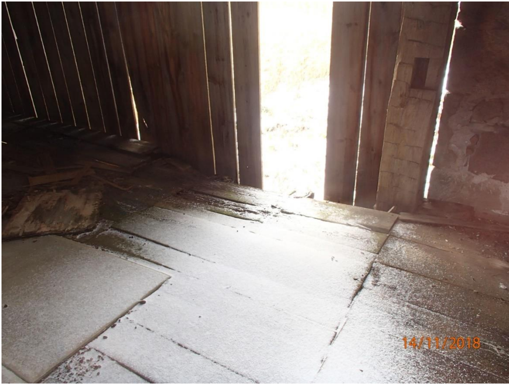
Photograph No. 13 – Condition of wall and floor in 2018
