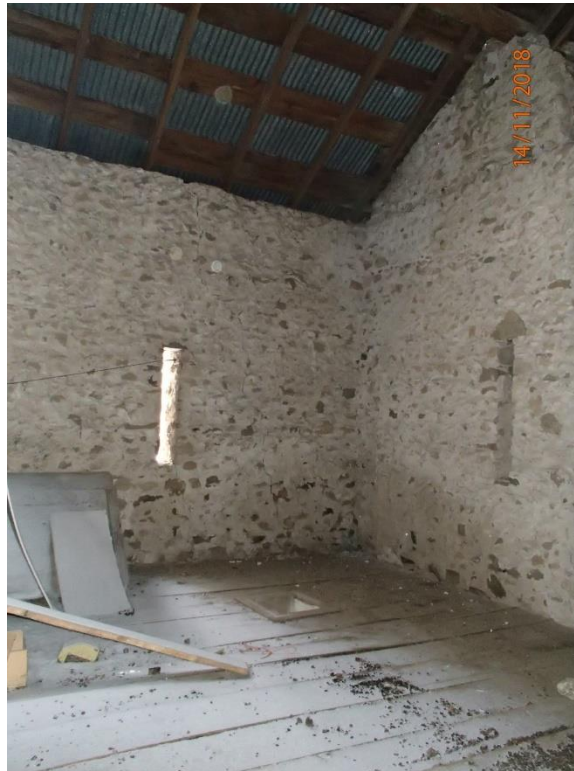
Photograph No. 9 – North wall (main floor) condition in 2018
