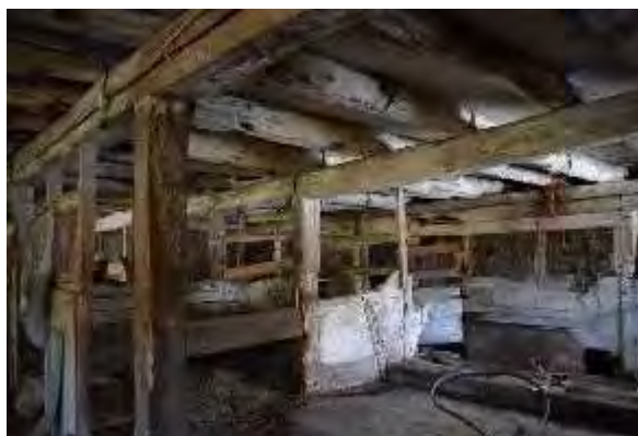
Plate 135: Horse stalls looking northwest
