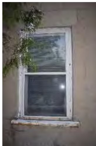
Plate 29: Wood 1/1 single-hung window on north elevation
