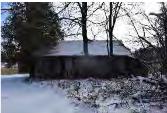
Plate 150: Outbuilding looking south
