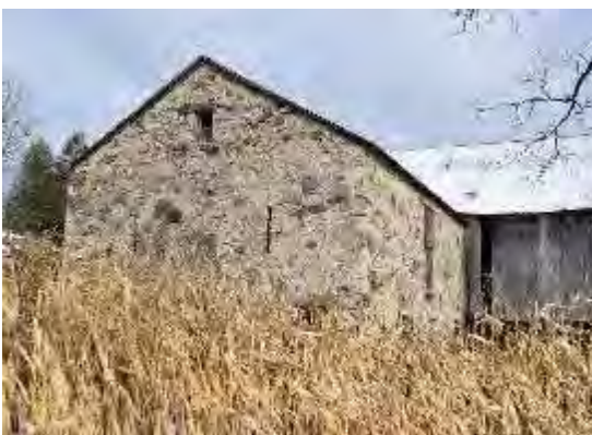
Plate 92: West elevation looking northeast
