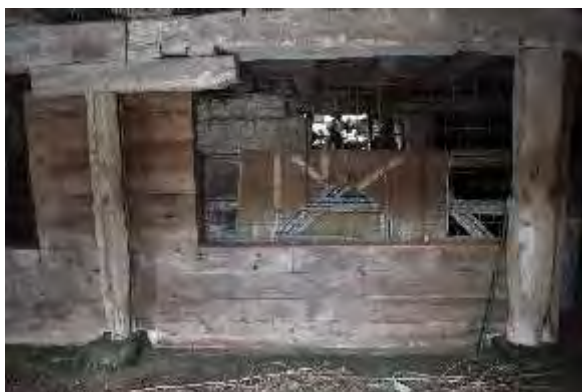
Plate 142: Hand hewn posts in stone tail on stones
