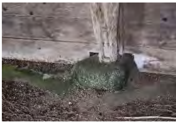
Plate 143: Close-up of stone supporting hand hewn beam
