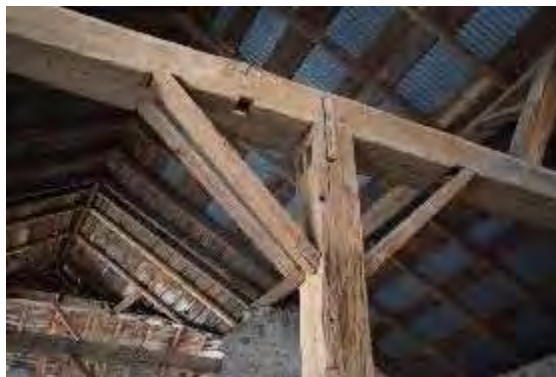
Plate 119: Close-up of stone tail post and beam joint
