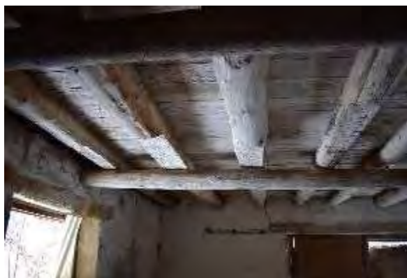
Plate 133: Old growth beams looking south
