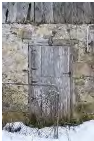
Plate 83: Wood door on east elevation
