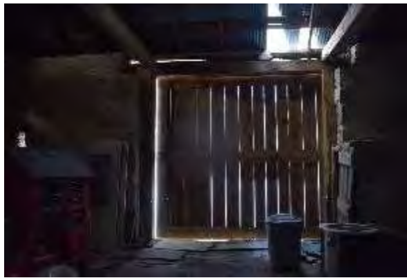
Plate 123: Wood frame entrance door looking north
