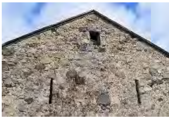
Plate 93: Gable peak of west elevation
