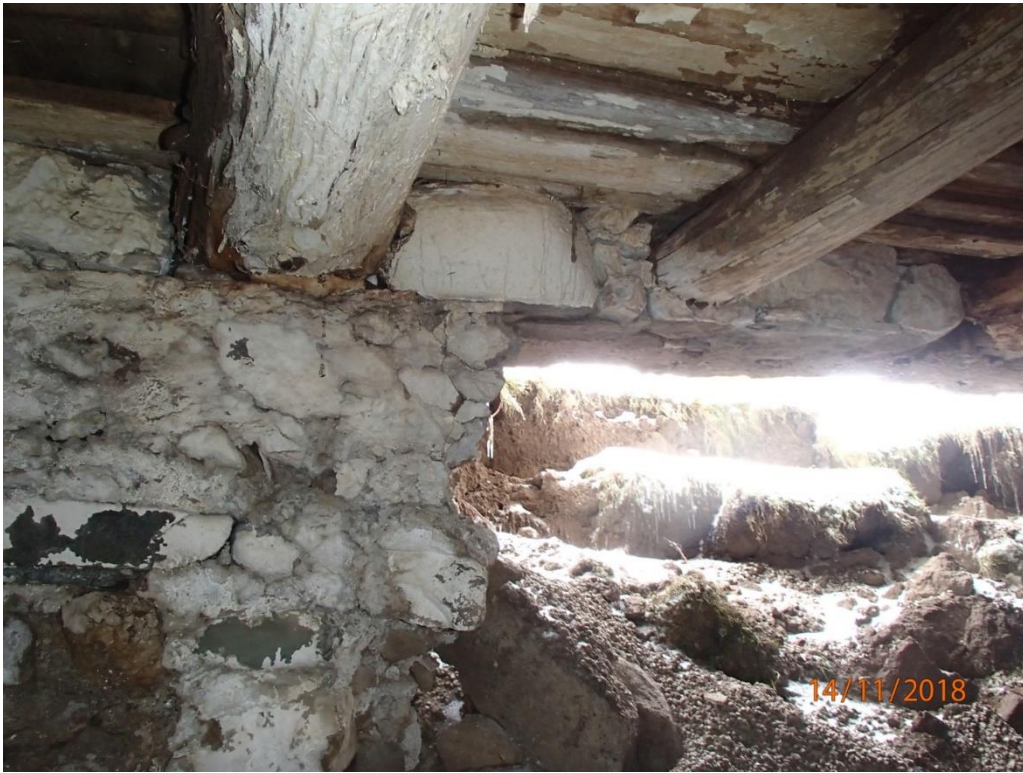
Photograph No. 5 – North wall (lower level – Left bearing) condition in 2018
