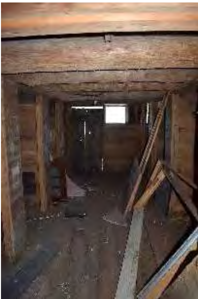
Plate 105: Enclosed grain storage area looking east
