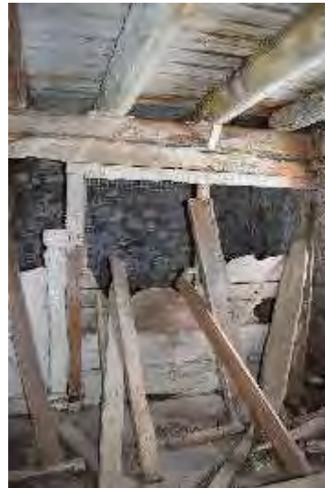
Plate 137: Horse stalls looking northeast
