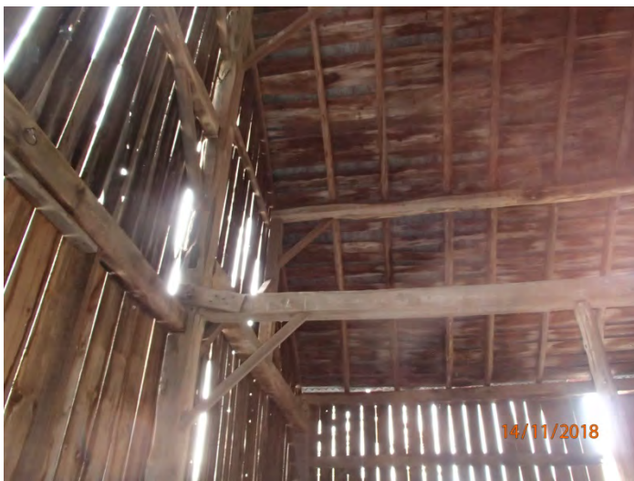
Photograph No. 13 – Superstructure barn roof framing (fair condition)
