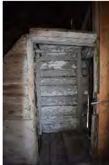
Plate 110: Wood vestibule to lower stables looking west
