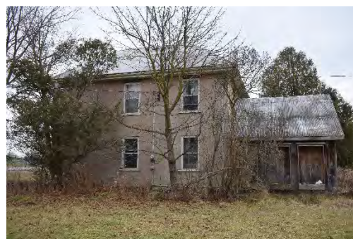
Photo 4-4: North elevation looking south
