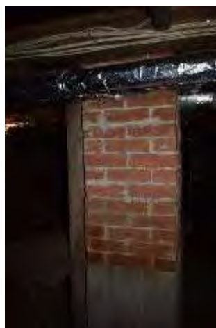
Plate 56: Interior brick chimney
