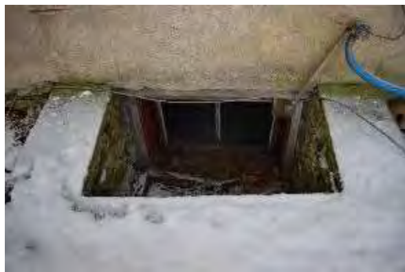
Plate 30: Stone window well on east elevation
