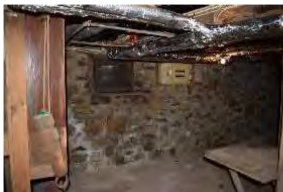
Plate 52: Basement looking northeast
