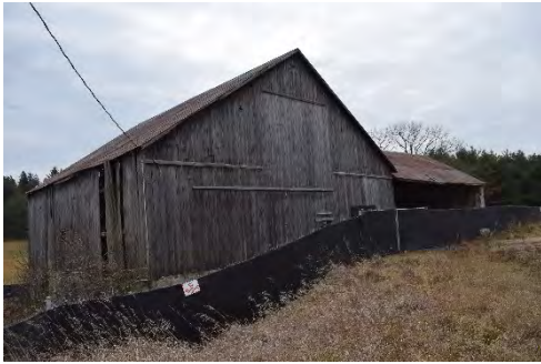
Photo 4-5: North elevation looking south
