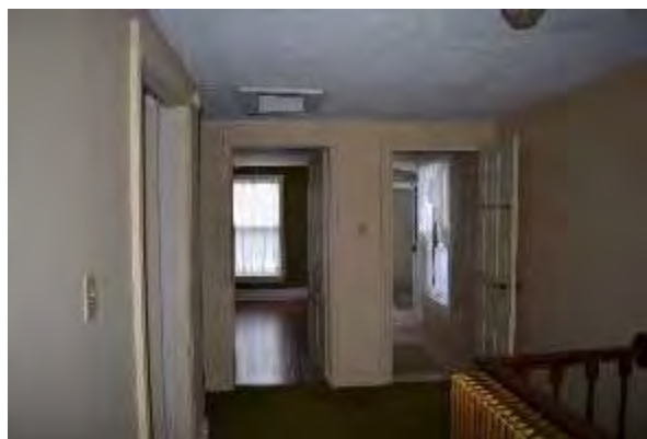
Plate 62: Central upstairs hallway looking south
