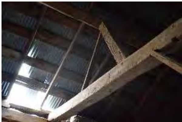
Plate 120: Stone tail beam and strut
