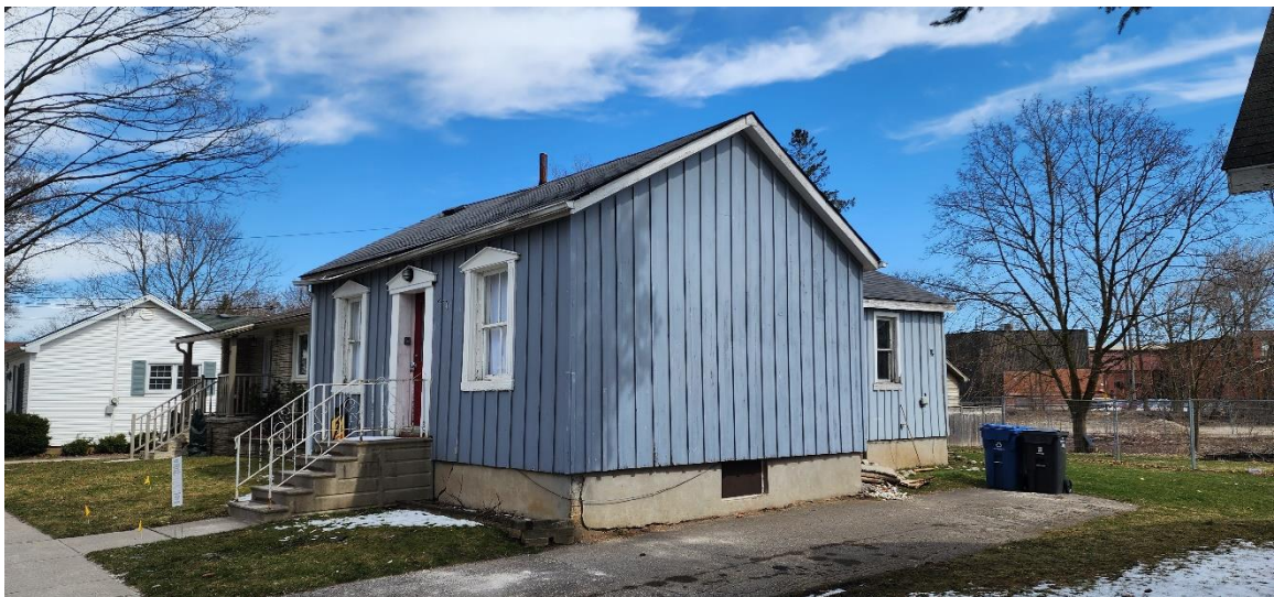
Figure 3 - 9 Omar St from north. (Photo: S. Robinson, Heritage Planning, City of Guelph, 2024)
