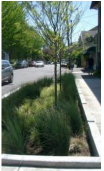
Low-Impact Development (LID) is an approach to managing storm water run-off at the source by replicating natural watershed functions. It uses simple, cost-effective landscape elements to capture, detain and treat storm water where it falls.
