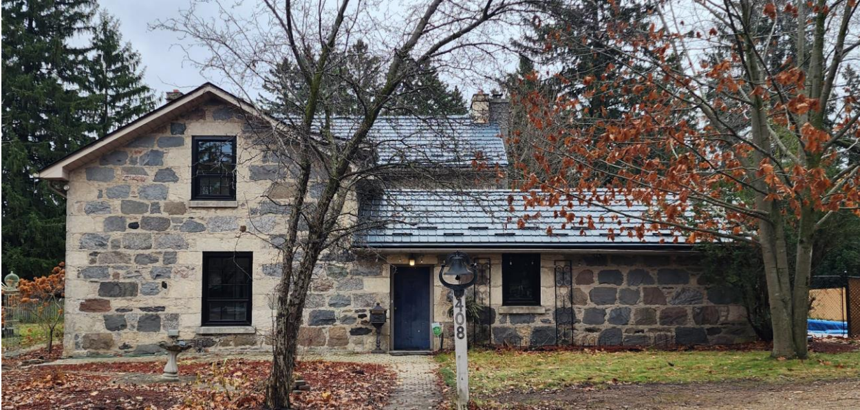
Figure 15 - North elevation of house. (Photo: S. Robinson)
