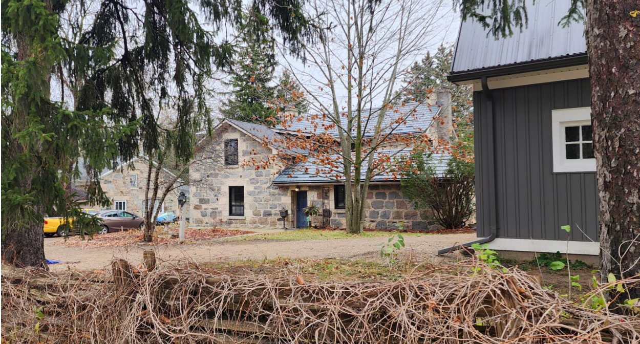
Figure 5 - House and garage from Willow Road. (Photo: S. Robinson)
