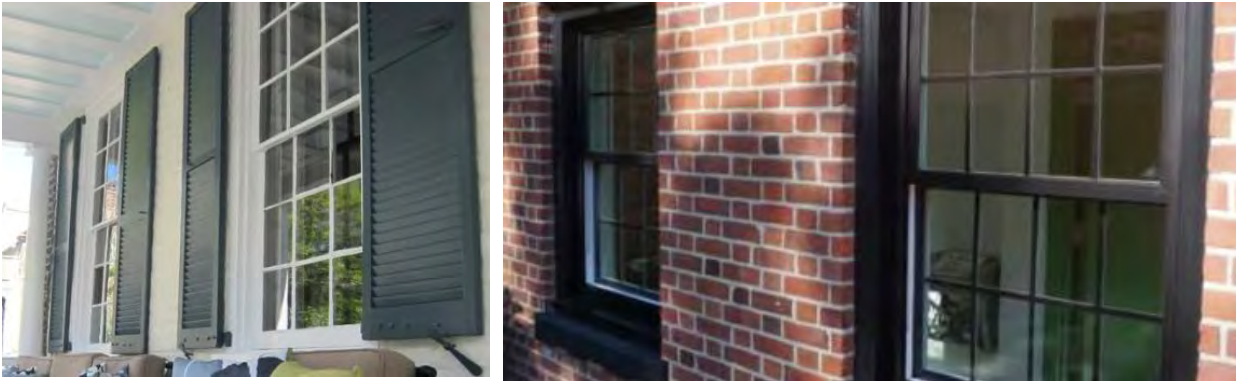
Figures 37 & 38: Samples of appropriate contemporary window designs for the Gothic Revival cottage style which include muntins. Other contemporary windows without muntins could also be used.
