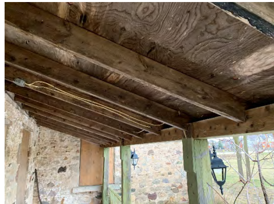
Photo 9: Underside of Covered Porch
