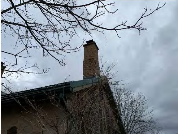
Photo 16: Summer Kitchen Brick Chimney
