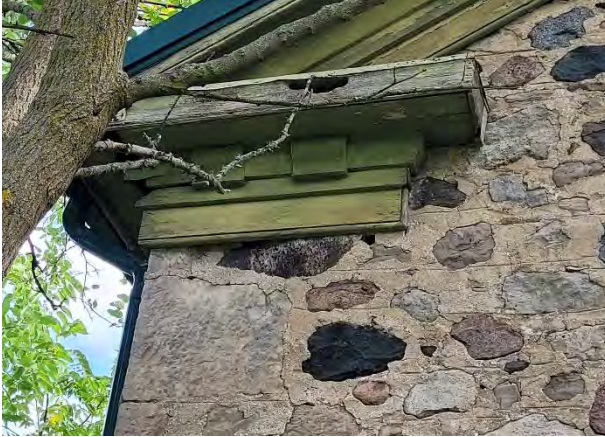
Figures 23 & 24: (left) Detail view of section of wood return eaves where wood is rotted, (right) Detail of wood eaves at the front elevation below the roofline (Source: MHBC, 2023)
