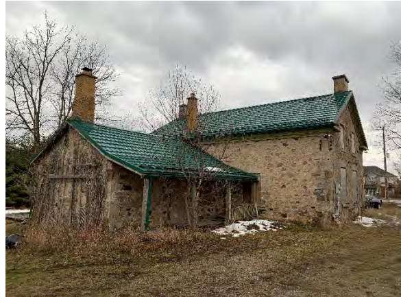
Photo 17: View of House showing all four chimneys
