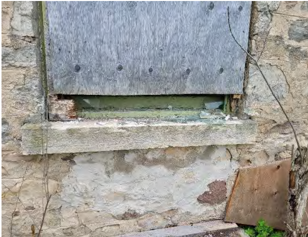
Figures 13 & 14: (left) View of north elevation, looking south (right) Detail view of broken window and sill at north elevation, (Source: MHBC, 2023)
