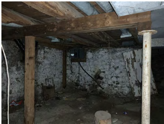
Photo 14: Typical Rubble Foundation Wall
