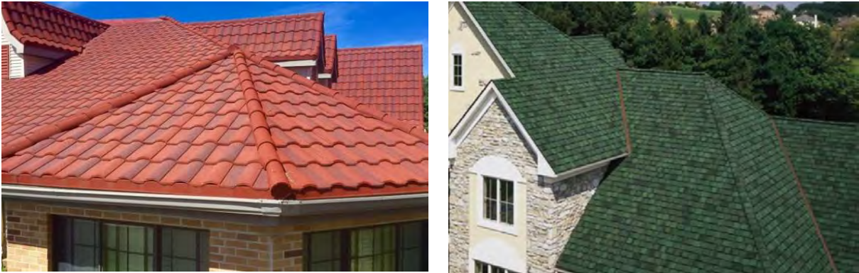
Figures 49 & 50: Samples of inappropriate contemporary materials, including vibrant terra cotta and coloured shingles which are not of a neutral colour palette.
