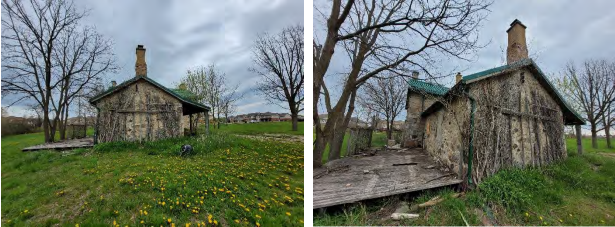
Figures 19 & 20: (left) View of east elevation looking west, (right) View of east and south elevations, (Source: MHBC, 2023)
