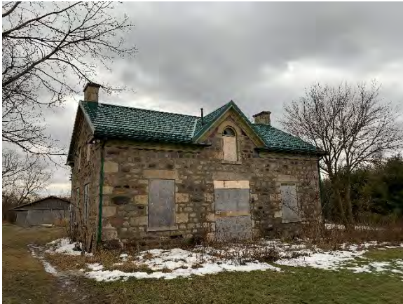
Photo 1: Main House (Principal Elevation -West)
