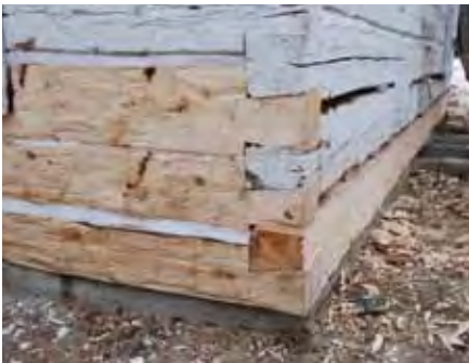
Deteriorated logs at the John Walter Historic Site in Edmonton were replaced in kind with hewn logs that used the originals as templates to reproduce tooling marks on visible surfaces. On close inspection, this distinguishes the new materials if the logs are separated in the future.
