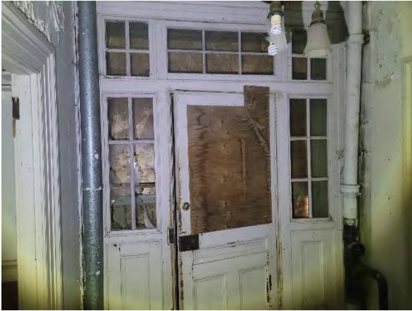
Figures 25 & 26: (left) View of interior of the building and central door opening at front elevation noting condition of wood frames and glazing, (right) View of typical first storey window noting broken glazing and condition of wood framing, (Source: MHBC, 2023)
