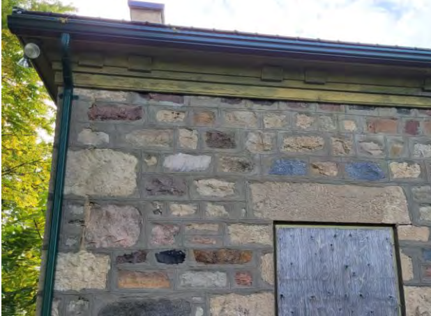
Figures 23 & 24: (left) Detail view of section of wood return eaves where wood is rotted, (right) Detail of wood eaves at the front elevation below the roofline (Source: MHBC, 2023)
