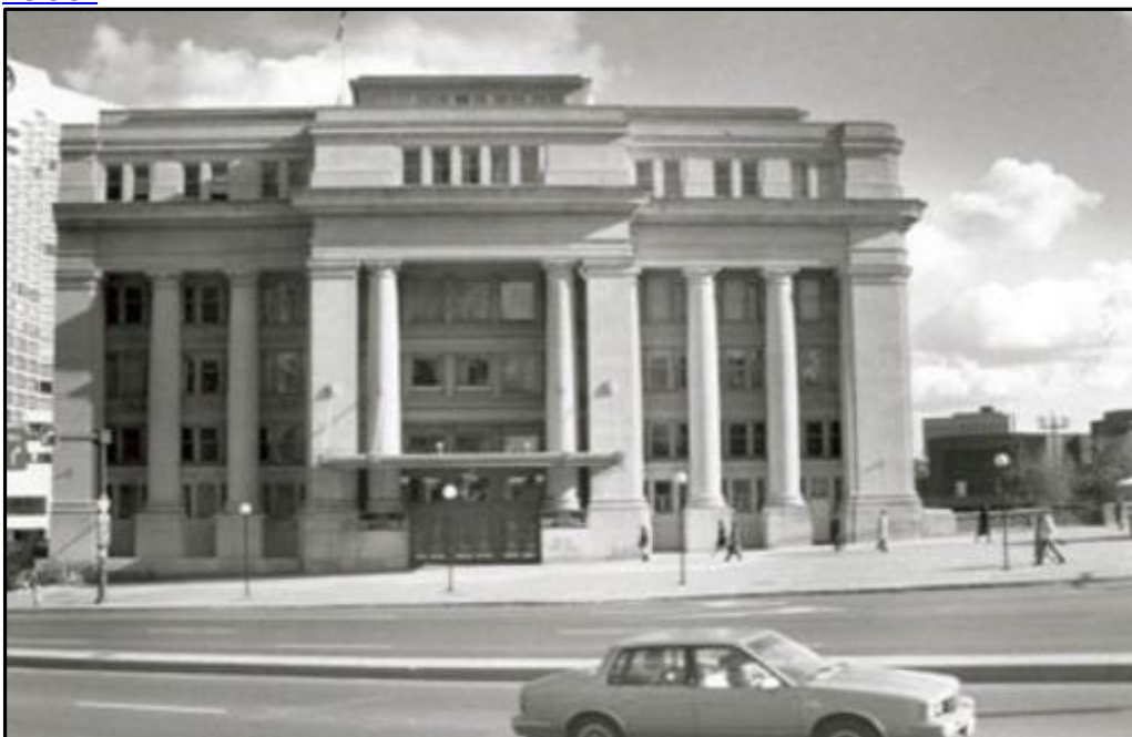
Figure 6: Former Union Station, now Government Conference Centre. Ottawa, 1988.
