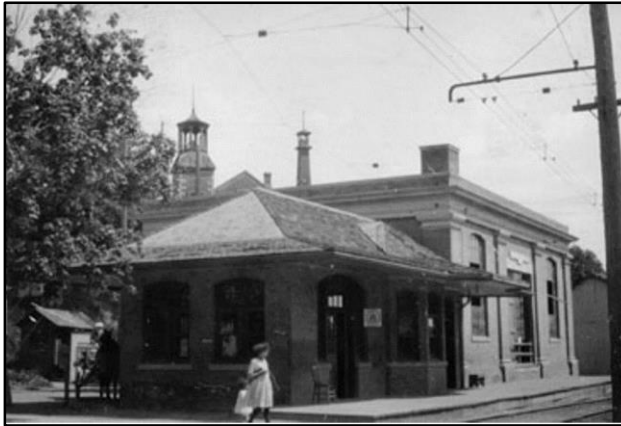
Figure 9: Georgetown TSR Station, Source: The Georgetown Vault .
