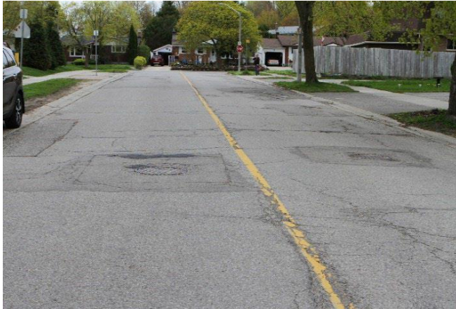
Figure 5: Condition Rating Very Poor (1>0)
