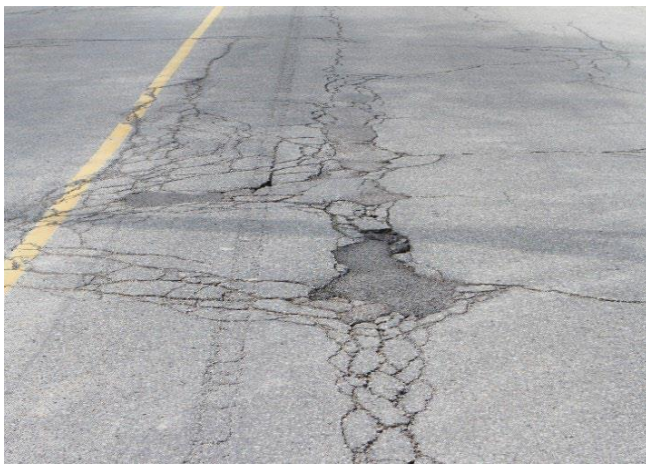
Figure 5: Condition Rating Very Poor (1>0)
