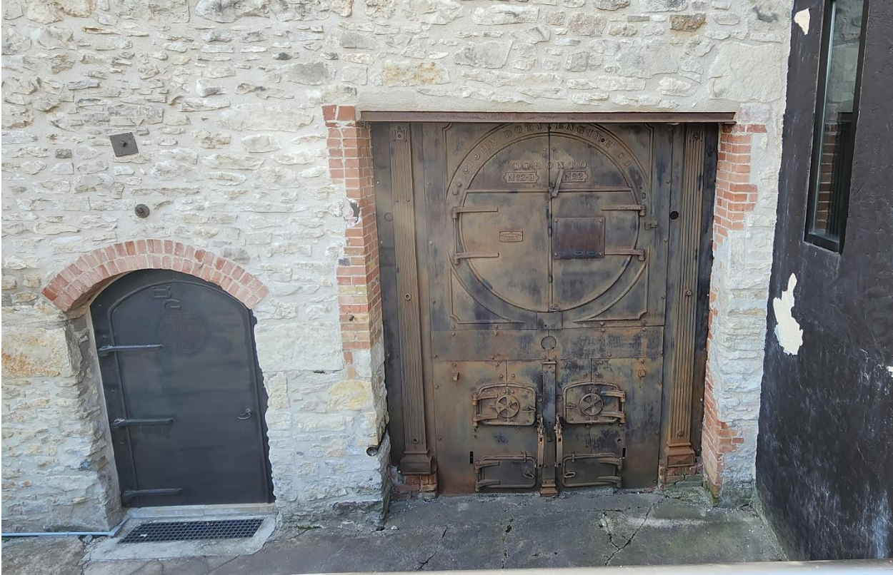
Figure 7 - Image of 167 Suffolk Street West, boiler doors (S. Robinson 2023).
