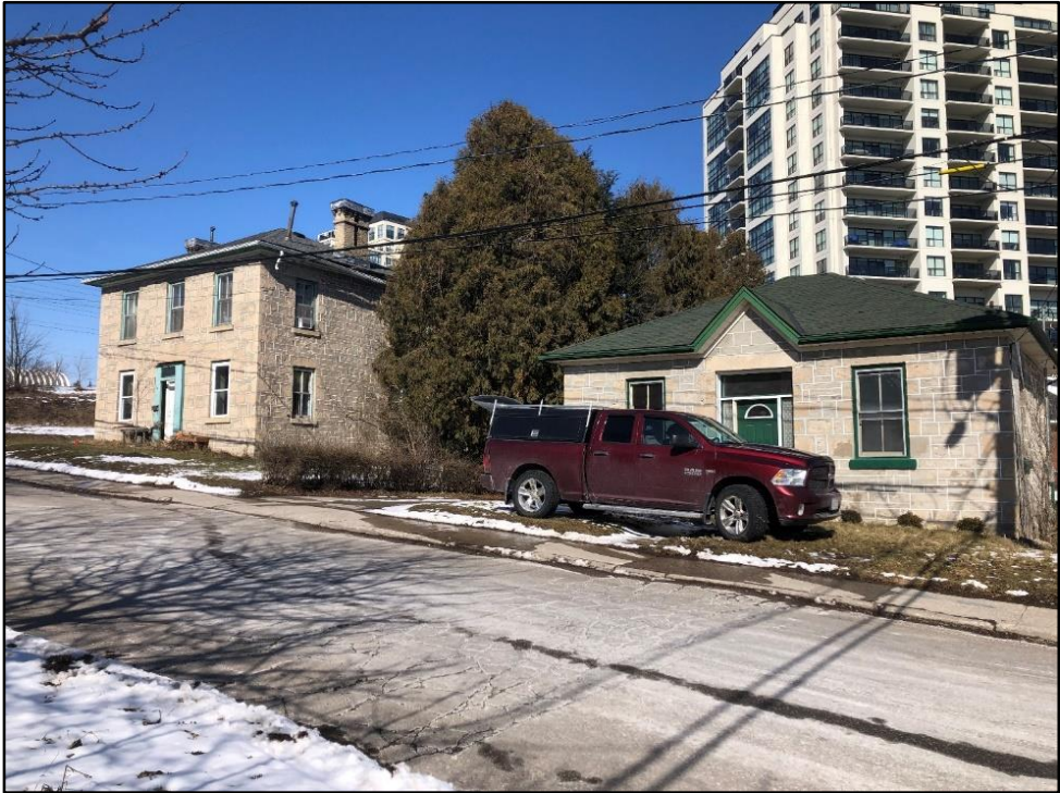
Figure 9: 14 Neeve Street and neighboring stone house, likely built around the same time and out of the same limestone.
