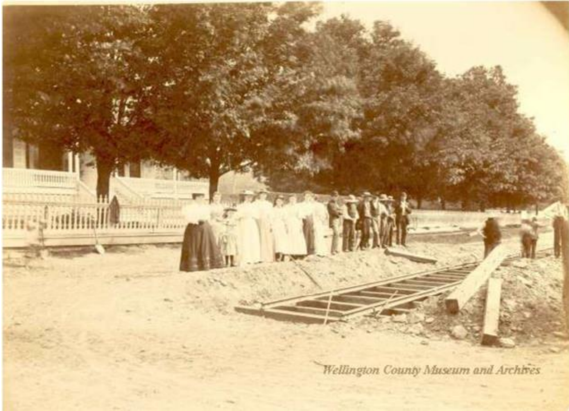
Figure 12 – Workmen laying streetcar tracks in front of the Sleeman House, c. 1900 (Wellington County Museum & Archives A1952.312.3B)
