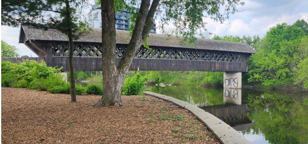
Figure 9 - View along wall to covered bridge. (Photos: S. Robinson, 2024)
