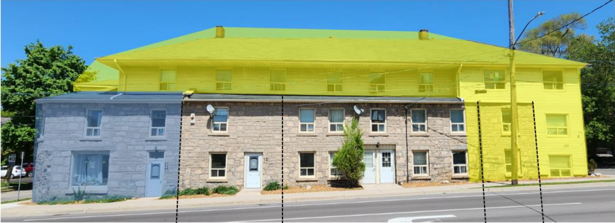
Figure 9 - Overlay on photo depicting the stages of construction. (Photo and overlay: S. Robinson, 2023)
