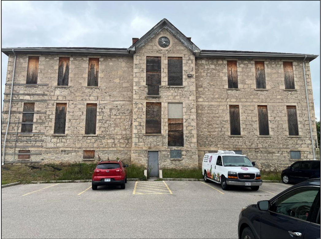
Figure 5: South elevation (heritage staff 2024)
