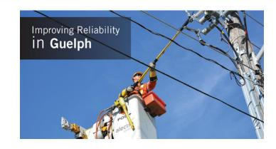
Focused on asset renewal and customer-driven work impacting 3,000 customers in Southwest Guelph – replacing underground cables and renewing overhead poles.
