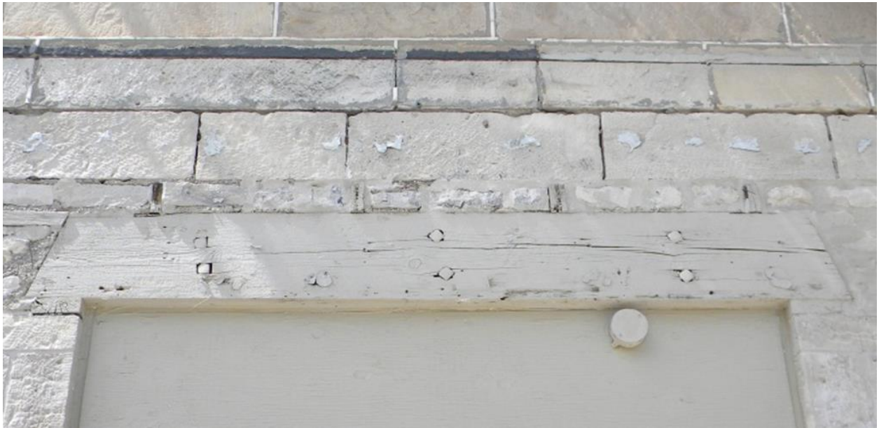
Figure 5 - Wooden lintel on main floor, possibly from the 1840's stable building. The opening is similar in size to the ones visible in the photographs from the 1880s. (Photo: S. Robinson, Heritage Planning)
