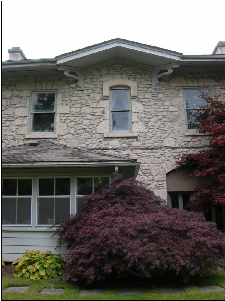
Figure 3: Enclosed Verandah and protruding gable with carved cornice and brackets. Source: Site Visit with Franco Valeriote, 2009.
