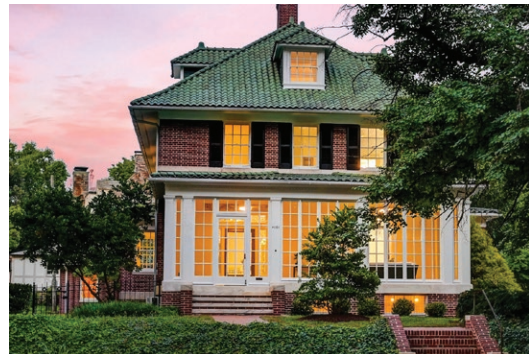
Wooden porch enclosure with white frames and mullions, Baltimore, Maryland (Photo by Eric Tyler).
