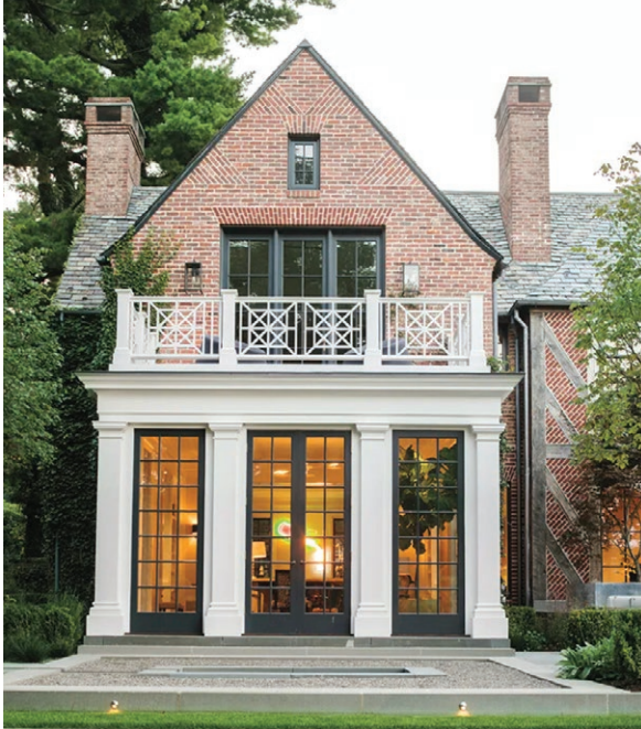
Porch enclosure set behind pilasters, with dark grey frames and mullions, Greenwich, Connecticut (Photo by Neil Landino Jr).
