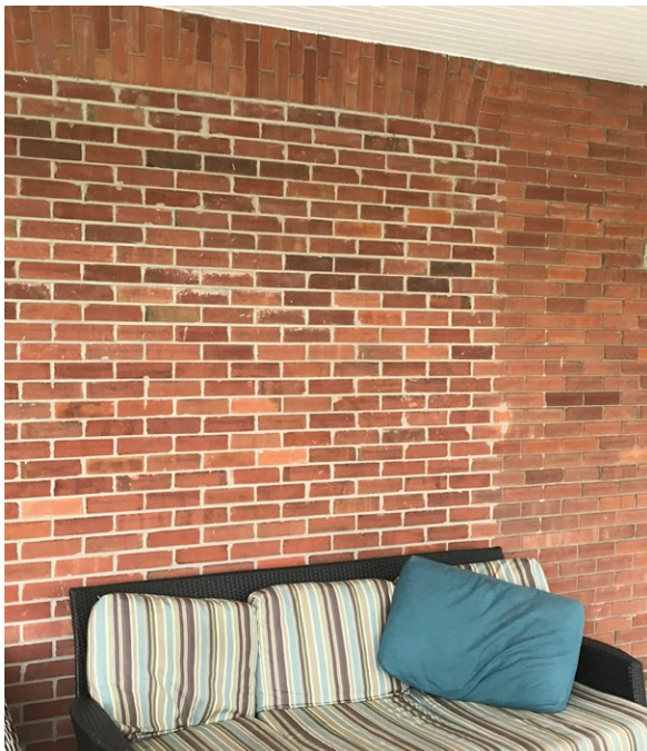
Masonry infill on ground floor of north portico (ERA, 2024).
