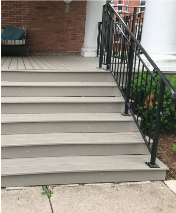
Existing stair and hand rail (ERA, 2024).
