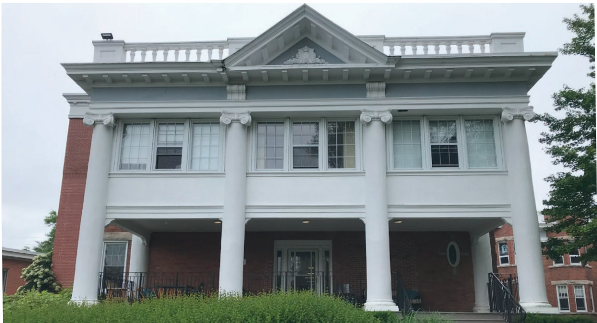
North portico, looking east (ERA, 2024).
