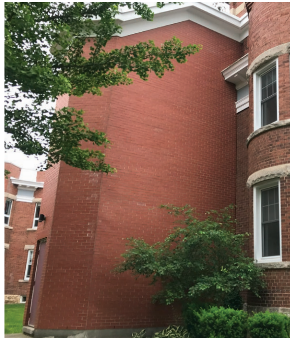
Stairwell D within north courtyard, looking east (ERA, 2024).
