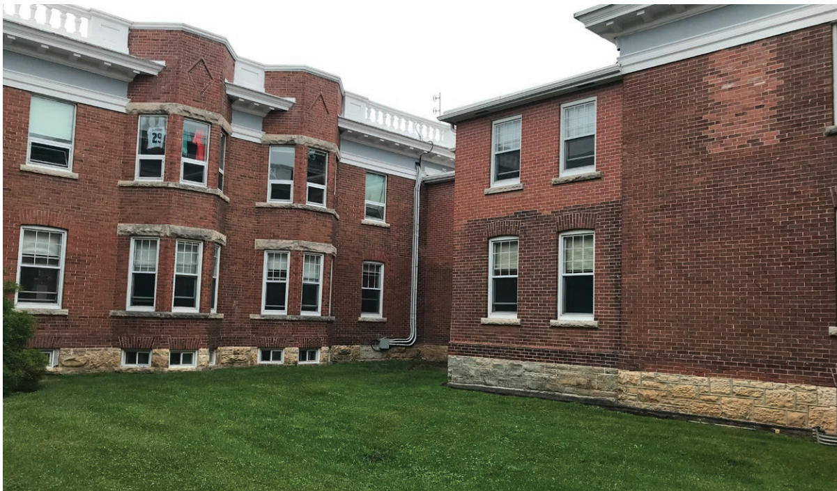
North courtyard, looking southeast (ERA, 2024).
