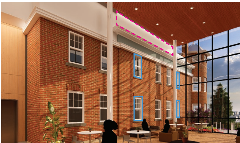
Rendering of proposed condition of central wing's north elevation, with reinstated windows outlined in blue and the removed balustrade outlined with a dashed pink line (Cornerstone, 2024; annotated by ERA).
