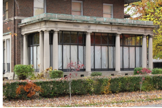
Residential porch enclosure set behind Doric columns, Detroit, Michigan (Photo by Scott Weir).
