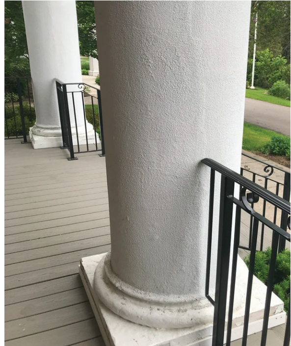
Close-up of north portico column and hand rail (ERA, 2024).
