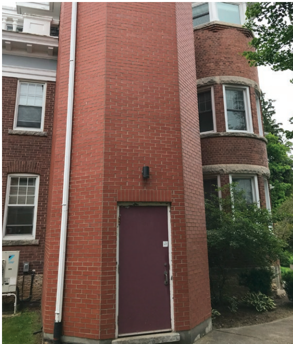
Stairwell D within north courtyard, looking south (ERA, 2024).
