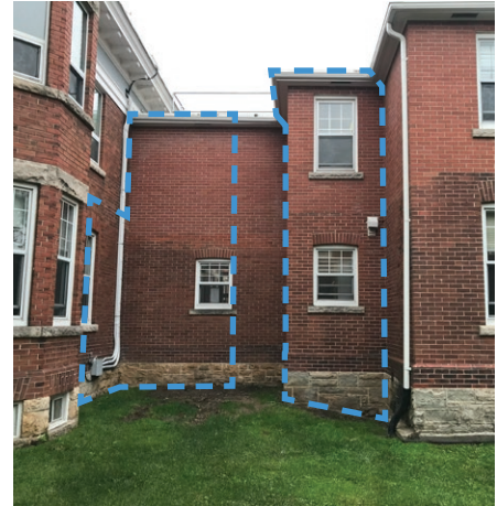
North courtyard indicating approximate areas of existing masonry to be removed outlined in blue (ERA, 2024).
