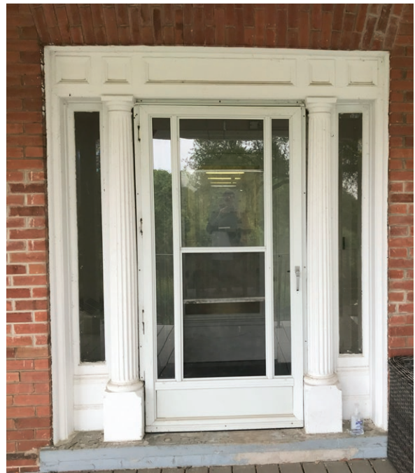
Entrance to north wing (ERA, 2024).
