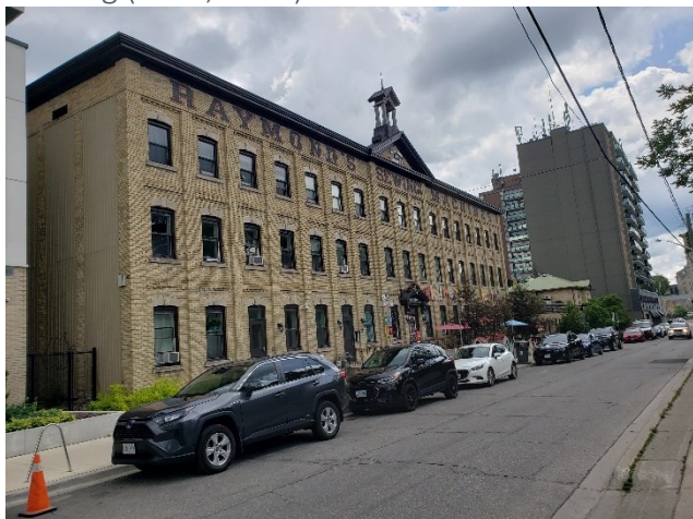
Figure 89: Looking southeast along on Yarmouth Street towards the Raymond Sewing Machine building (A.S.I., 2023).
