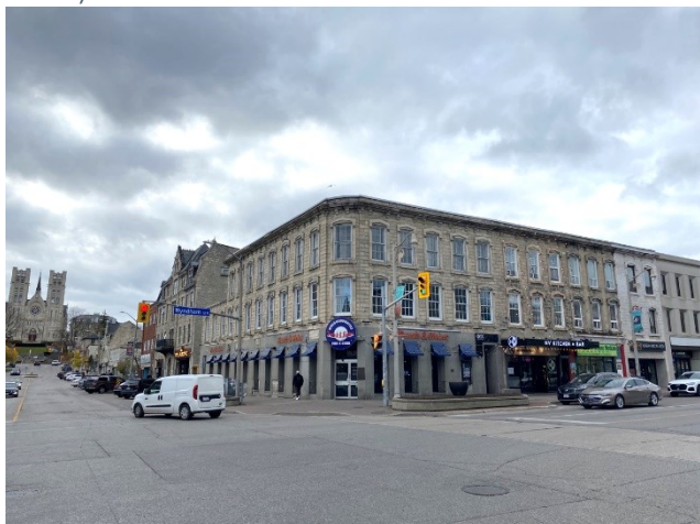
Figure 83: Elliott Block at 16-20 Wyndham Street North, constructed circa 1859-1860 (A.S.I., 2023).
