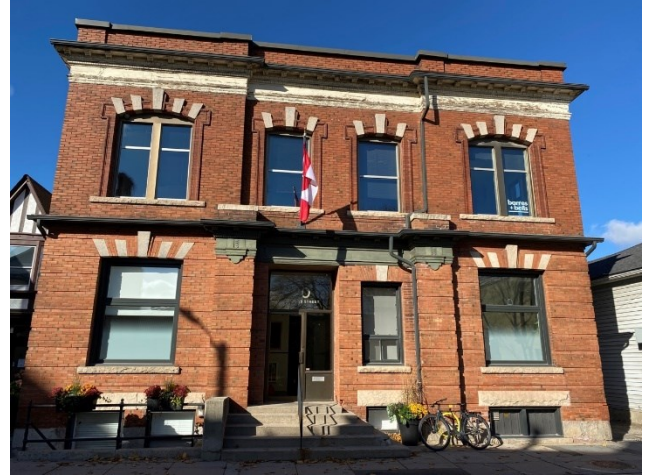
Figure 70: Red brick building at 30/32 Douglas Street (A.S.I., 2023).
