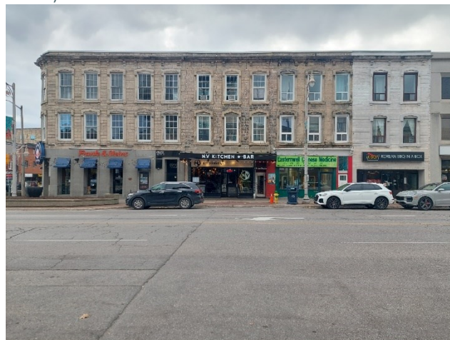
Figure 84: Elliott Block at 16-20 Wyndham Street North, constructed circa 1859-1860 (A.S.I., 2023).
