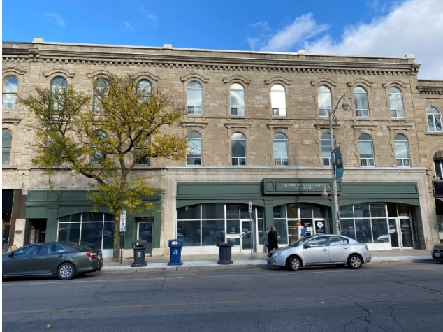
Figure 69: Limestone building at 137-145 Wyndham Street North (A.S.I., 2023).
