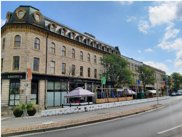
Figure 50: Wyndham Street, looking southeast from Woolwich Street (A.S.I., 2023).
