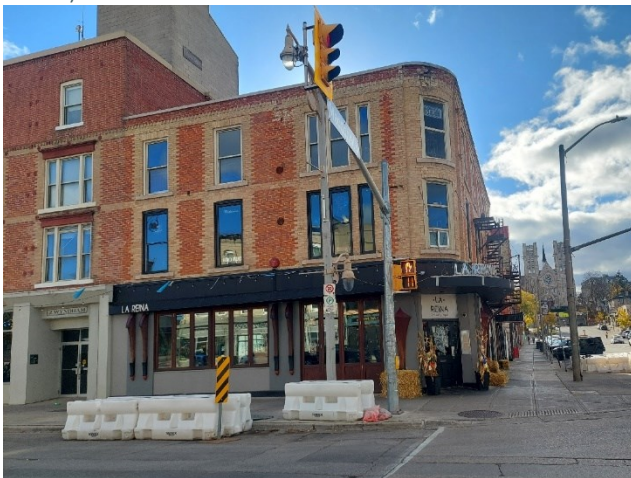
Figure 73: 8-10 Wyndham Street North (A.S.I., 2023).
