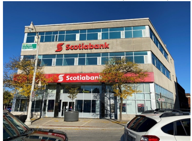
Figure 64: 83 Wyndham Street North, constructed circa 1960s-1970s (A.S.I., 2023).
