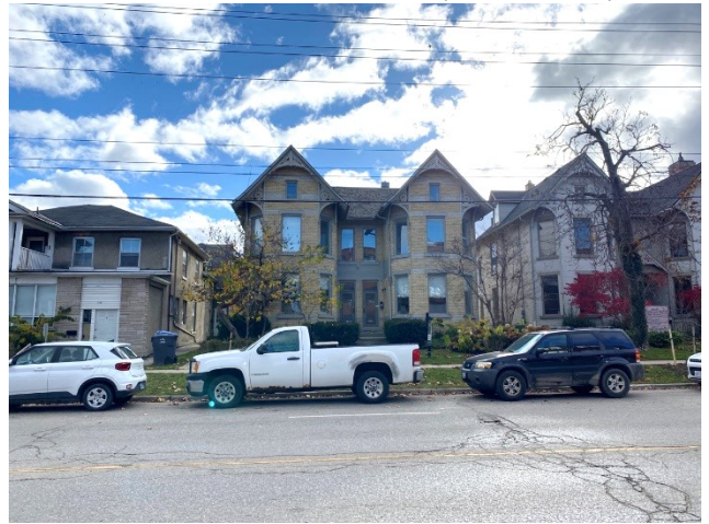
Figure 68: A row of residential properties on Woolwich Street, some of which have been converted for commercial use (A.S.I., 2023).
