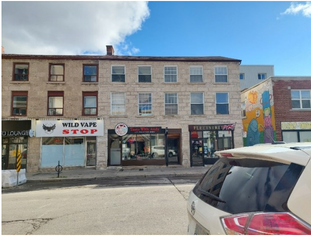
Figure 87: 45 Cork Street East, designed by William Day (A.S.I., 2023).
