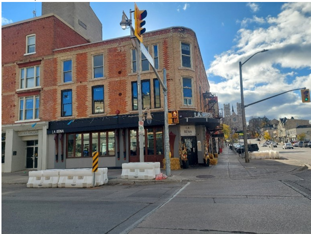
Figure 71: 8 -10 Wyndham Street North (A.S.I., 2023).
