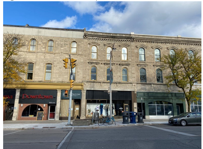
Figure 72: 128 - 133 Wyndham Street North
