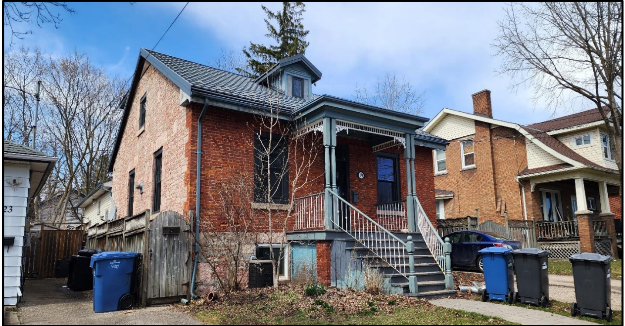
Figure 1 Photograph of 19 Fountain Street West, left of center.
