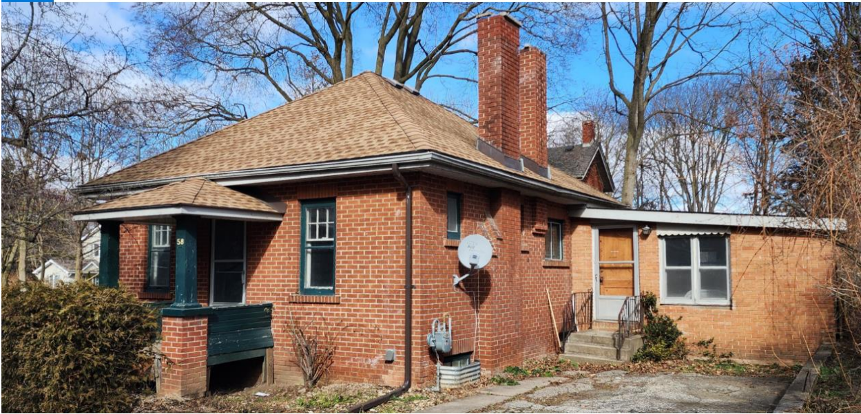
Figure 7 - View of house from south.
