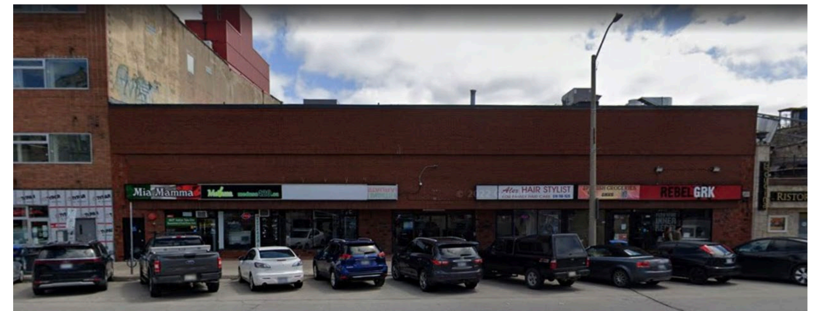
Figure 3: Existing Building viewed from MacDonnell
