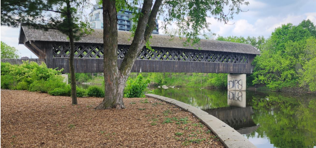
Figure 11 - View south along wall.(Photos: S. Robinson, 2024)
