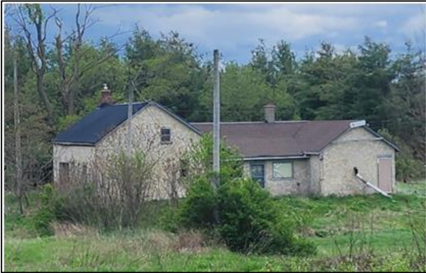
Figure 5 - Original roughly squared stone quoins revealed in northwest corner. (Heritage Planning 2024).
