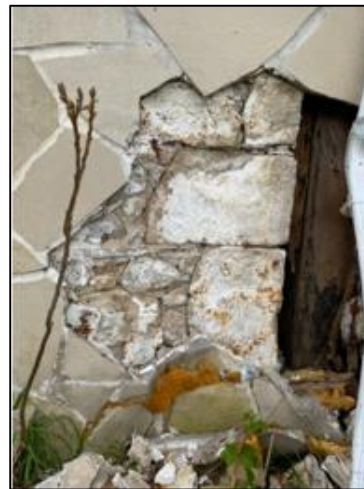
Figure 8: Roughly squared stone quoins, Northwest corner (Heritage Planning 2024).
