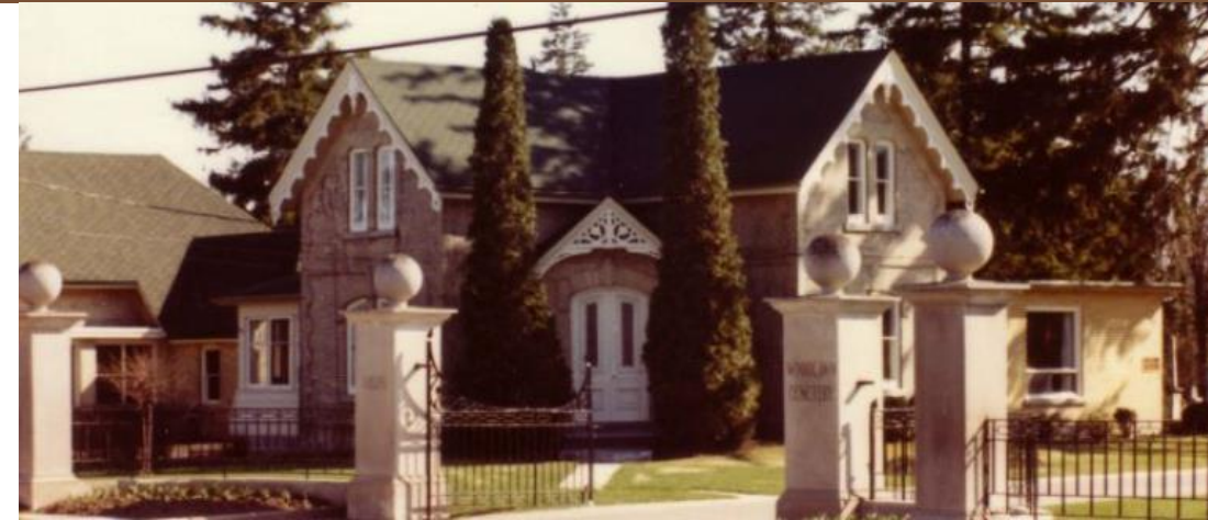
Woodlawn Memorial Park, Entrance Gates and Residence
