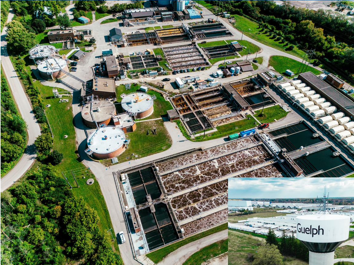
📍 Water Resource Recovery Centre
