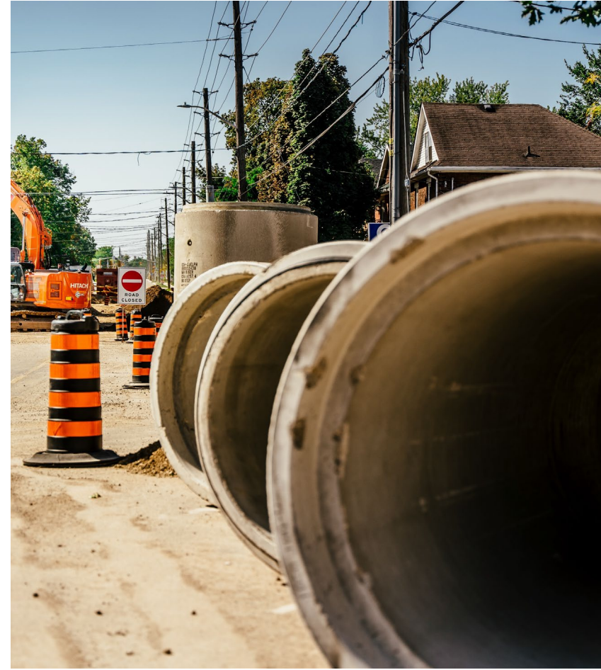
📍 A Guelph construction site
