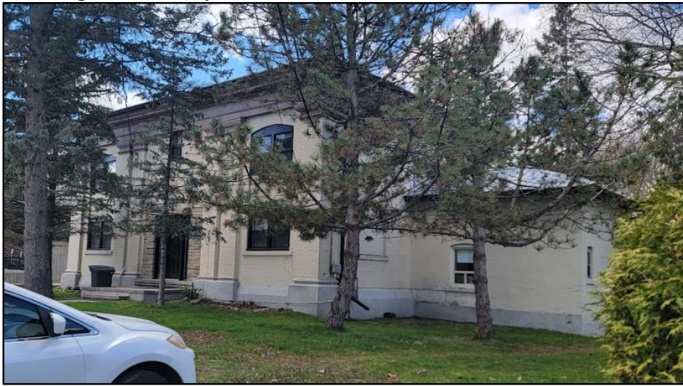
Figure 2: Photograph of the southeast corner of 22 James Street East (Heritage Planning Staff 2024)
