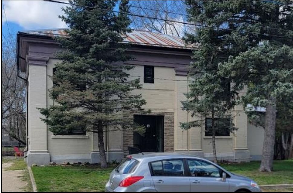
Figure 1: Photograph of the façade of 22 James Street East (Heritage Planning Staff 2024)
