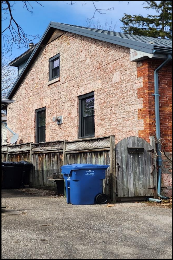
Figure 4: Western façade of 19 Fountain Street West
