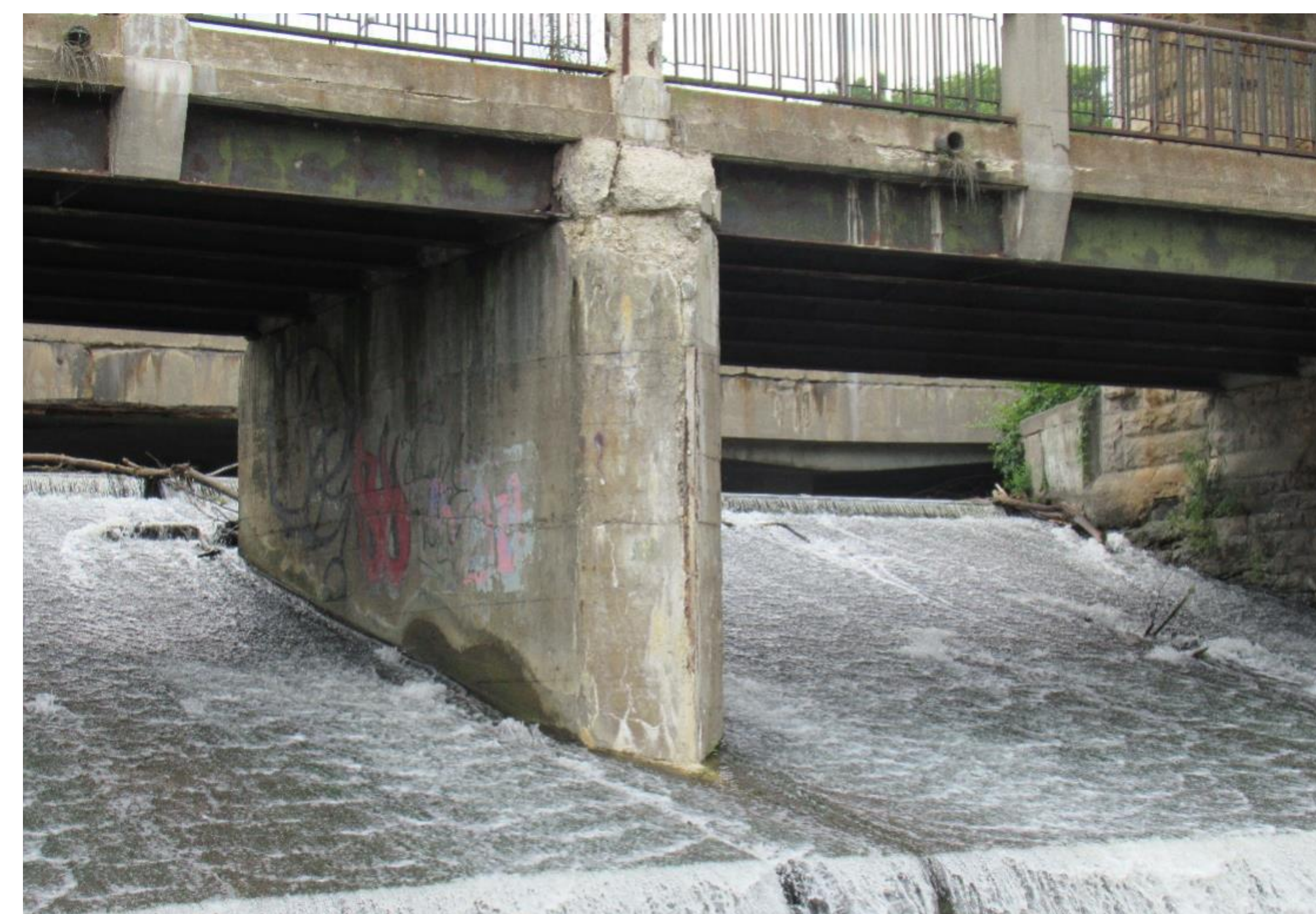
The spillway forms a weir to control the Speed River elevation, previously used for the now-removed Allan's Mill.
