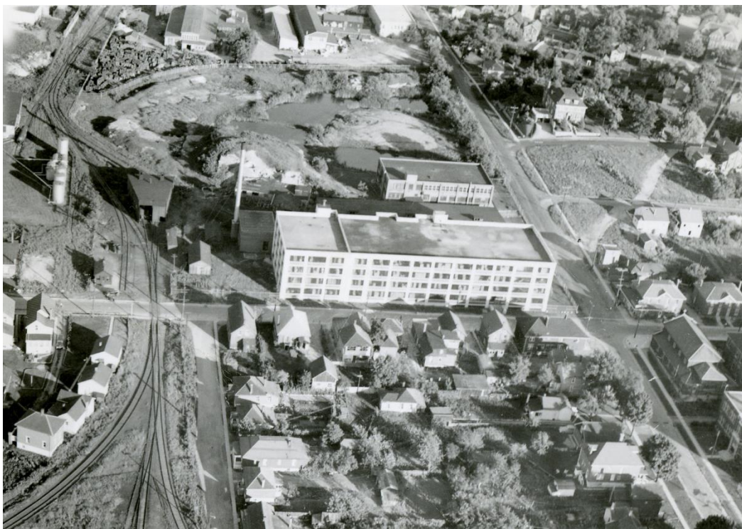
Spur line of the Guelph Junction Railway running parallel to Huron Street and crossing Alice Street (Guelph Museums 2014.84.608)
