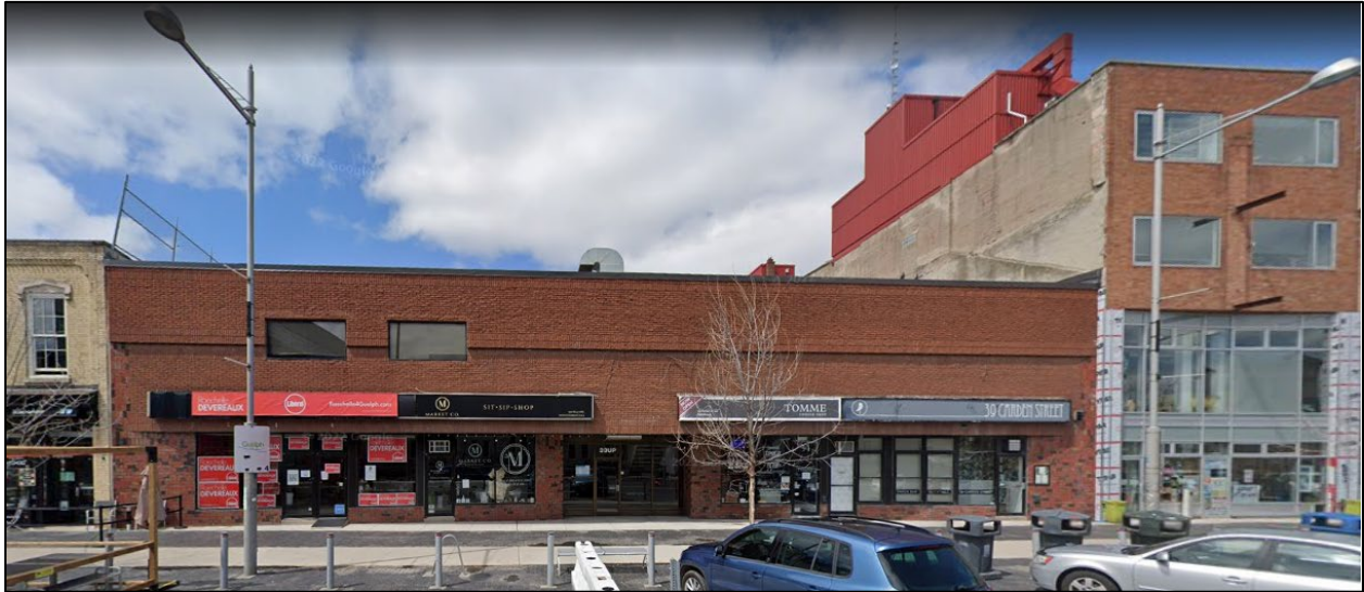
Figure 2: Existing Building viewed from Carden Street (Source: Google Streetview)
