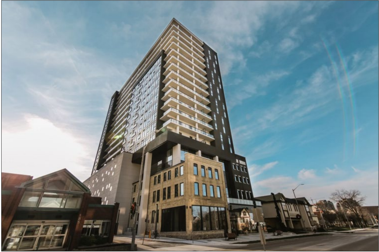
Figure 8: 181 King Street South, Waterloo
