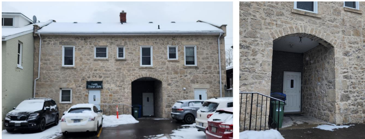
Figure 6 - Rear of building and carriage way arch. (Heritage Planning 2025)
