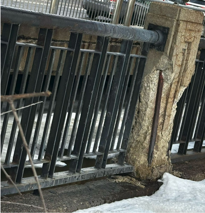
Figure 32 Feb 2025 Note rail pattern and posts similar to Michigan R4
