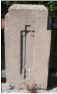
Figure 30 Michigan R4 Railing-first Generation Post
