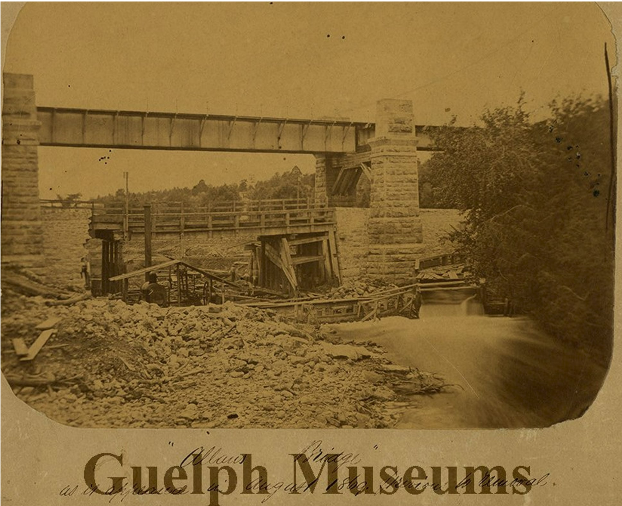
Figure 17 Image is labelled 1869 Aug. As it appeared prior to removal. This may be inaccurate since the wooden railway girders and braces were replaced in 1867. Note also the stone fill used for the abutments and what appears to be erosion of the west side abutment. The bridge is supported by a temporary posts on the west and cribbing on the east. This would be consistent the 1869 flood... more research is needed to establish the date with certainty.
