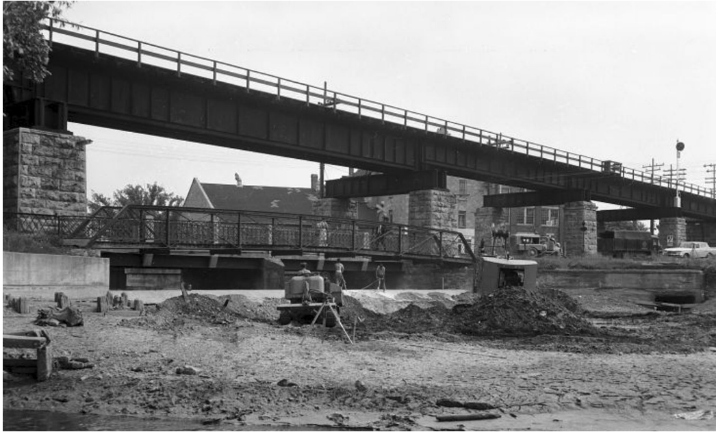
Figure 38 1963 MacDonnell St Bridge under construction
