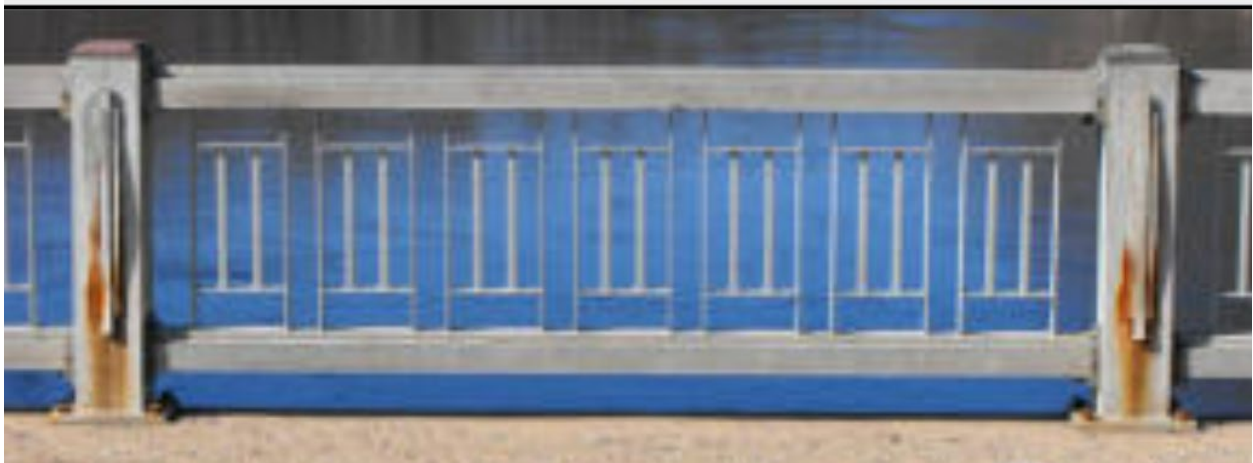
Figure 30 Michigan R4 Railing-first Generation Post
