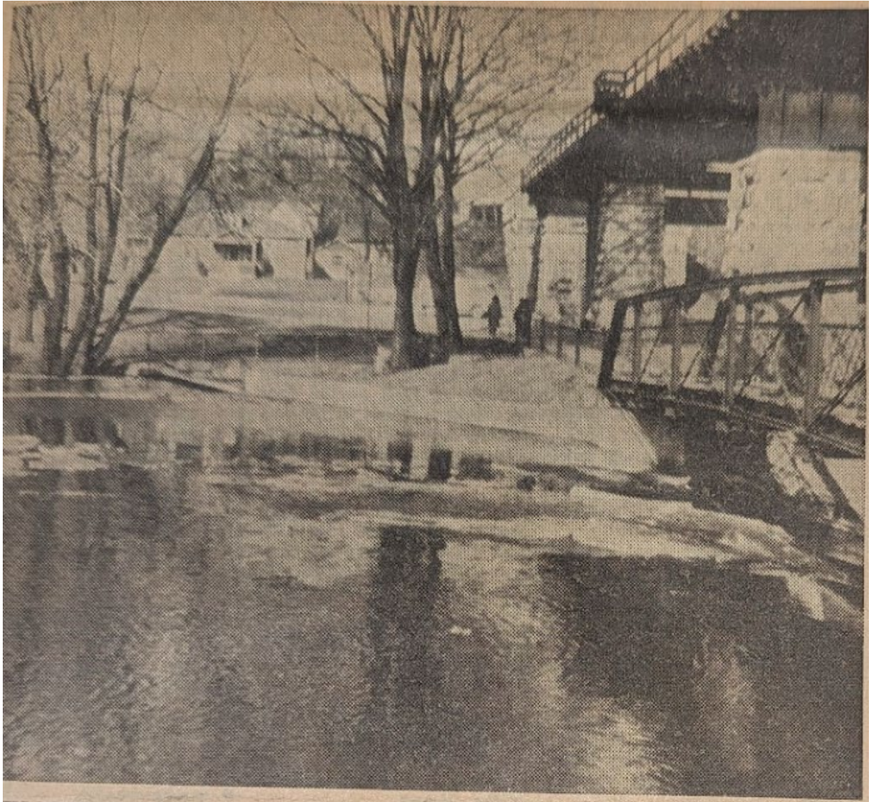
Figure 35 1962 Guelph Mercury before MacDonell St Bridge
