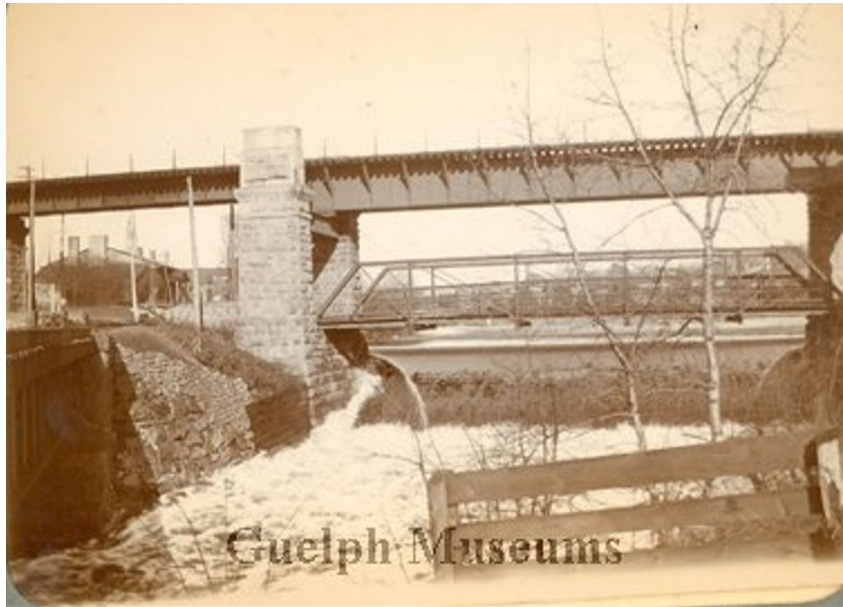
Figure 26 1903 Photo -Iron bridge as constructed (1892), Iron girders under viaduct (1867), and Guelph Junction Railway Bridge (1887) Note absence of centre support.
