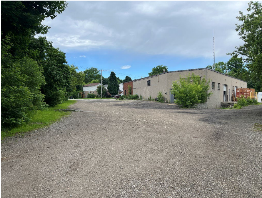
Plate 18: View of an industrial building on a large lot that fronts onto Dufferin Street (A.S.I., 2024).
