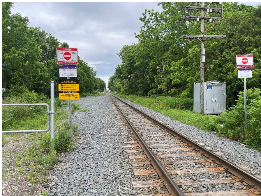
Plate 27: Guelph Junction Railway tracks at the south end of the C.C.H.L. (A.S.I., 2024).
