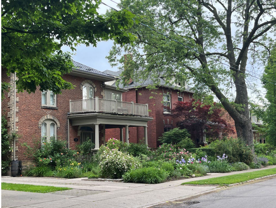
Plate 22: Row of houses along the northeast corner of Glasgow Street North and Liverpool Street (A.S.I., 2024).
