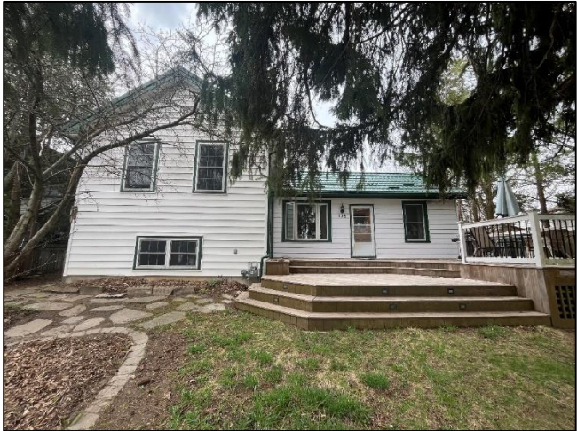
Figure 2: Facade of 128 Dufferin Street (Heritage Planning Staff, 2025)
