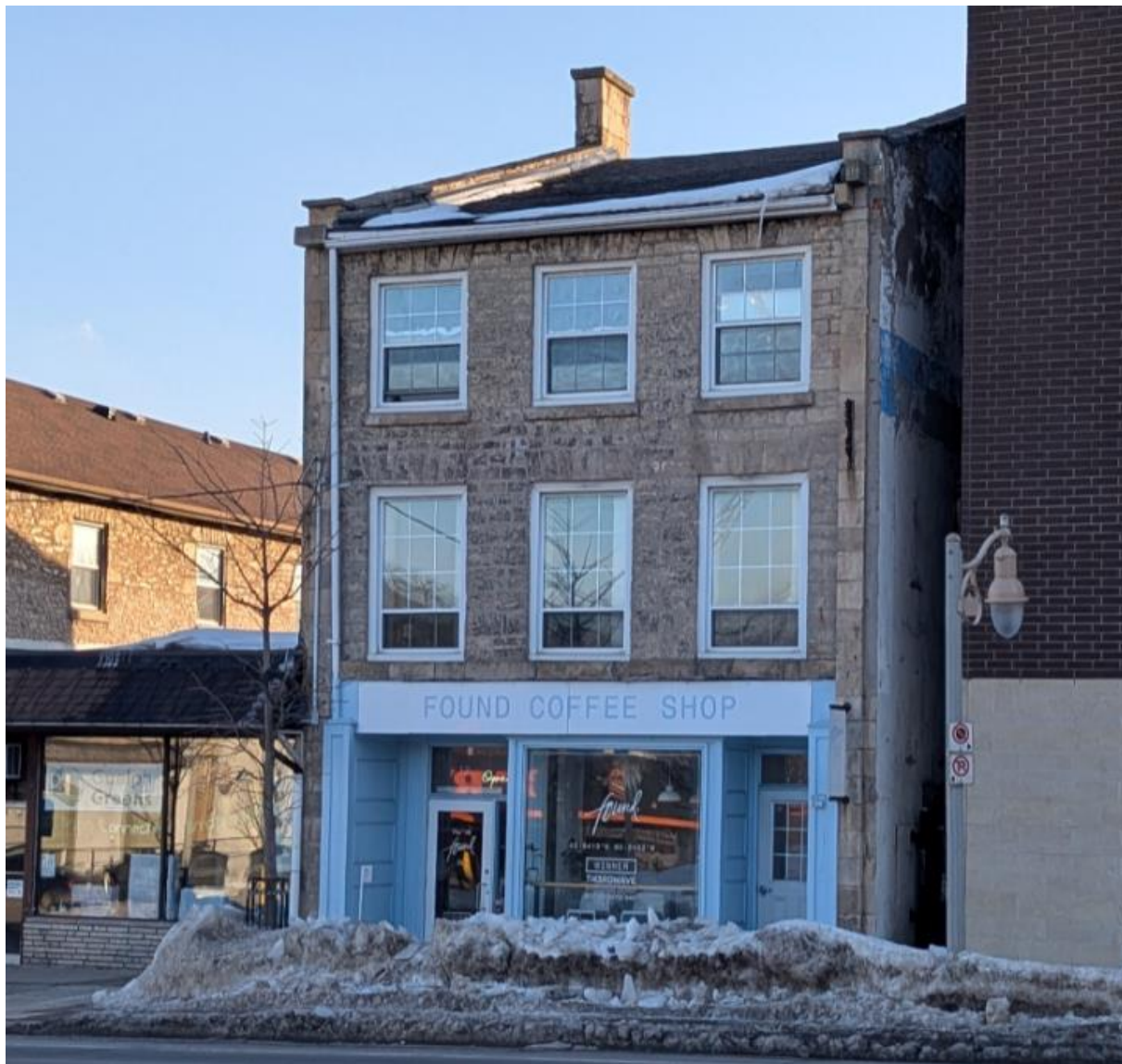
Figure 3 Current photo of 15 Gordon St. (Imogen Goldie, 2025)
