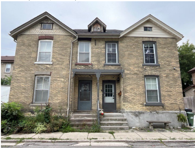
Figure 94: Buff brick cladding on 15-17 Oliver Street (A.S.I., 2024)
