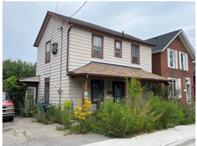
Figure 96: Vinyl siding on 44 Manitoba Street (A.S.I., 2024)
