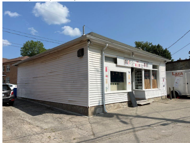
Figure 91: Commercial building at 72 Ontario Street (A.S.I., 2024)
