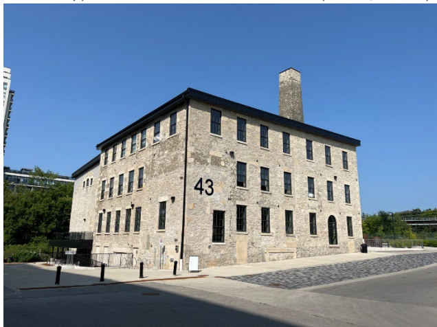
Figure 88: Industrial building (now the Spring Mill Distillery) at 43 Arthur Street South (A.S.I., 2024)
