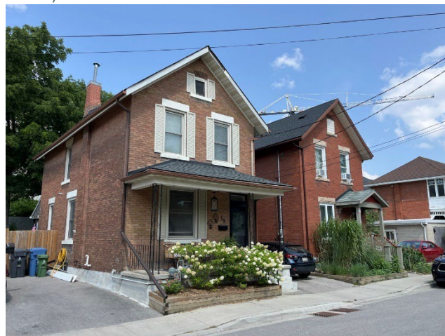
Figure 101: 58 and 60 Howitt Street, typical brick residences in a vernacular expression (A.S.I., 2024)
