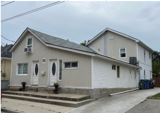
Figure 31: 134 Alice Street today, converted back to a residential use (A.S.I., 2024)
