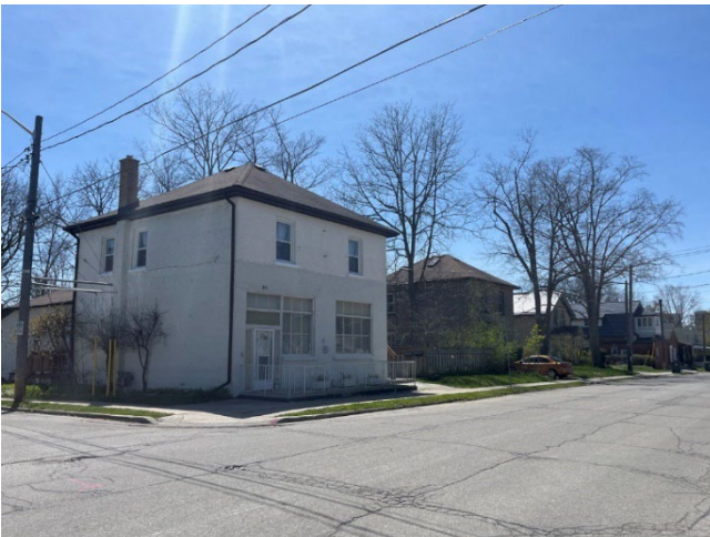
Figure 98: Mixed-use commercial/residential on Ontario Street at Short Street
