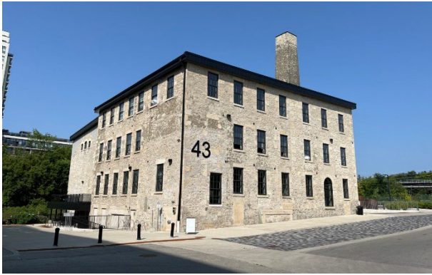
Figure 38: Remnants of Taylor-Forbes foundry adaptively reused as part of the re-development of the former industrial site (A.S.I., 2024)
