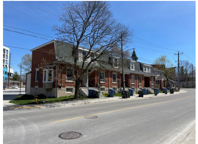
Figure 99: Rowhouses on Neeve Street
