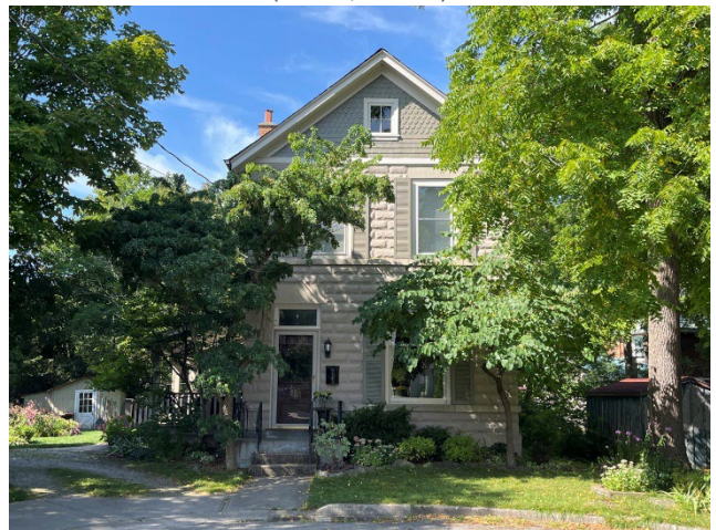
Figure 97: Concrete block cladding on 1 Richardson Street (A.S.I., 2024)
