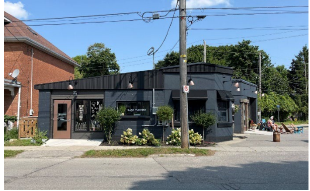
Figure 36: Former gas station at the corner of Ontario Street and Arthur Street South converted into several local establishments (A.S.I., 2024)
