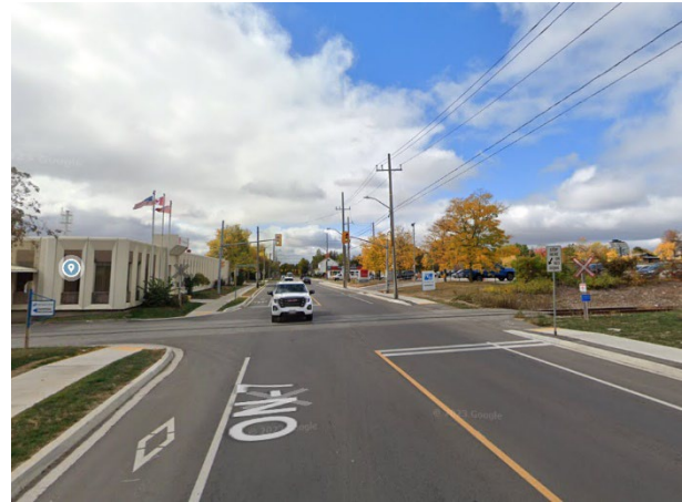
Figure 57: York Road and Guelph Junction Railway spur gateway (Google Streetview, 2022).
