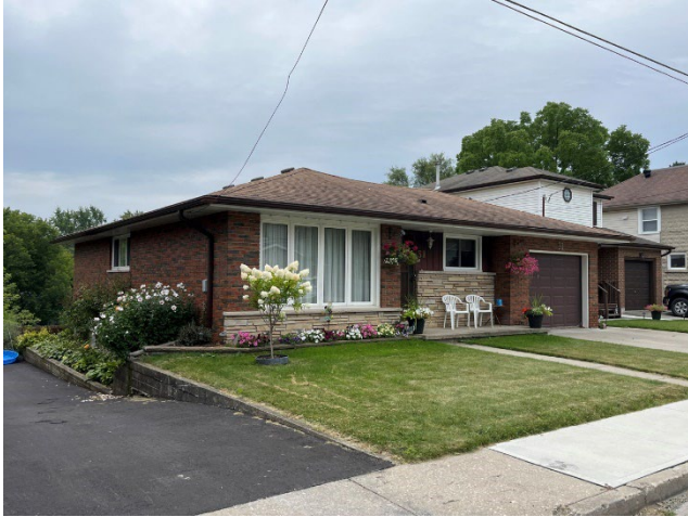
Figure 83: 31 Richardson Street, constructed circa 1960 (A.S.I., 2024)
