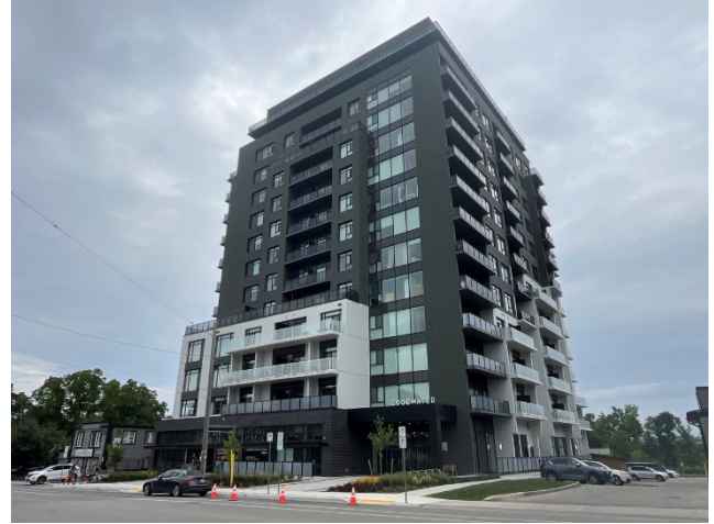
Figure 84: 71 Wyndham Street South, construction complete 2022 (A.S.I., 2024)
