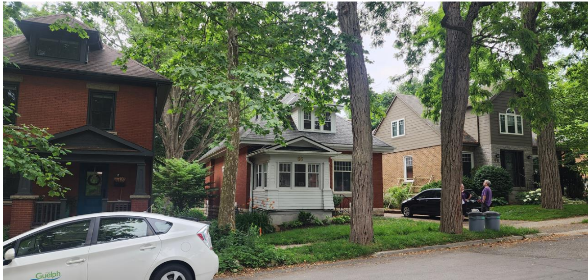
Figure 2 - View of 66 Mary St between adjacent properties (62 Mary St and 68 Mary St).
