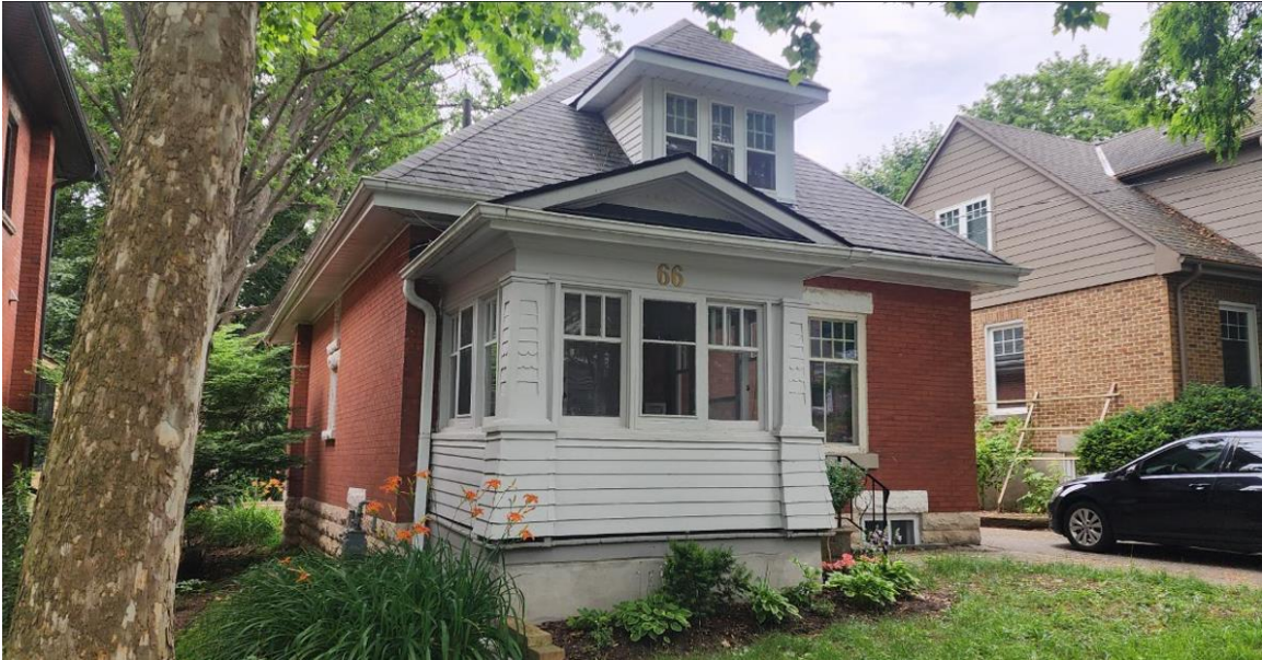
Figure 4 - 66 Mary St seen from west.
