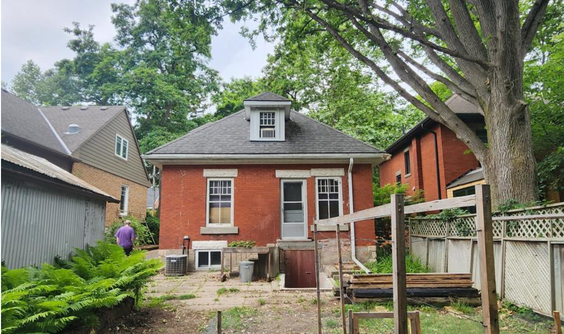
Figure 5 - 66 Mary St from rear yard with garage on left and large mature tree on right.
