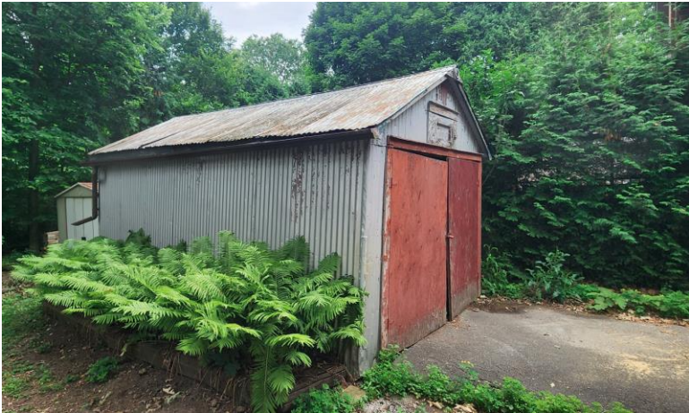
Figure 6 - 66 Mary St detached, metal-clad garage.
