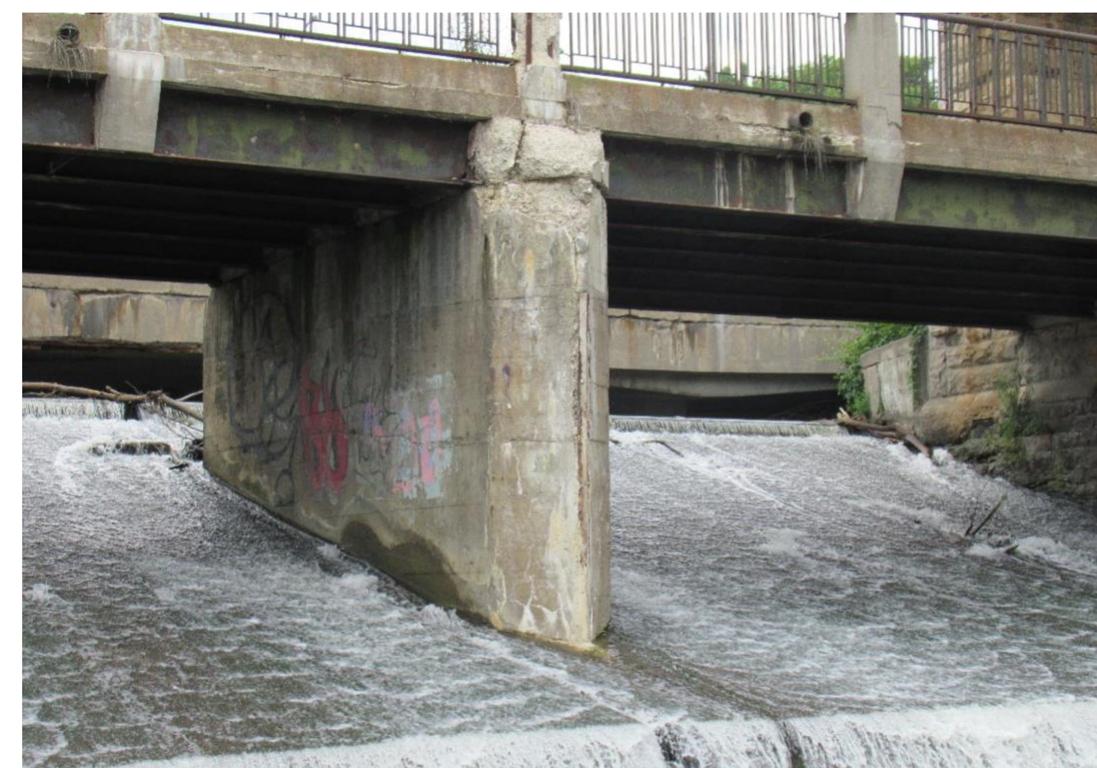
The spillway forms a weir to control the Speed River elevation, previously used for the now-removed Allan's Mill.
