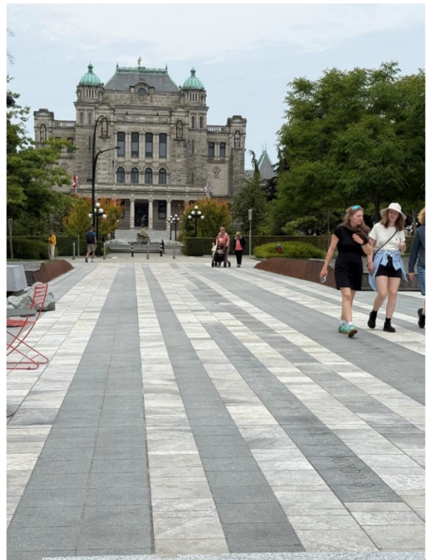
Figure 51: More accessible pavers at Capital Park in Victoria, British Columbia. The surface is lightly textured, low-glare, and the pattern is not visually overwhelming. The blocks are tightly jointed and define separate spaces for circulation and furnishings (Mark Steele).
