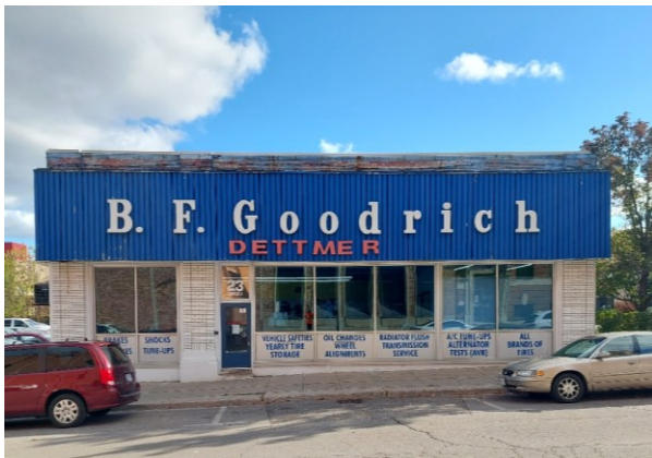
Figure 27: Dettmer Tire building with current cladding (A.S.I. 2023).
