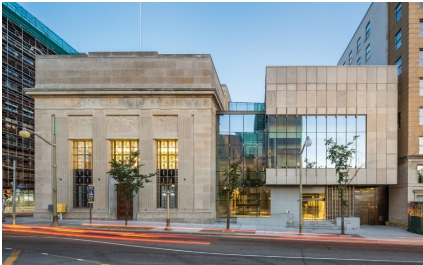
Figure 35: Example of addition to heritage building using visually and physically consistent material (stone) on the primary structure of the exterior wall, and contemporary cladding (glass) on the secondary structure of the exterior wall. Address: 144 Wellington Street, Ottawa (Doublespace Photography, 2015).
