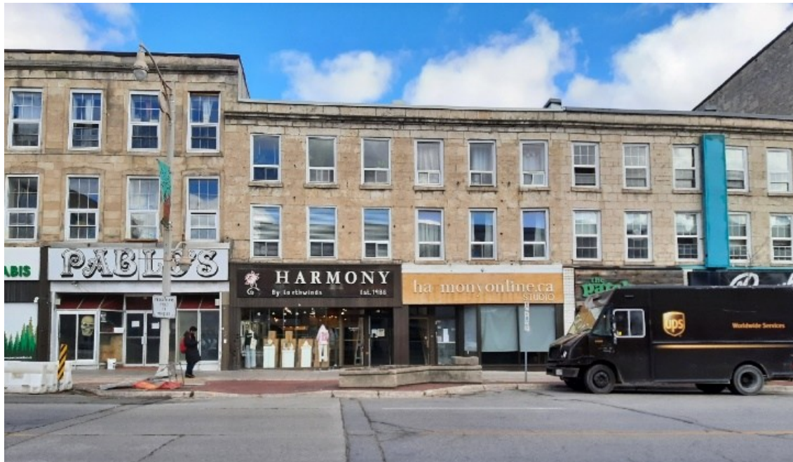
Figure 19: Stone buildings form the Wyndham Street streetwall , south of St. George's Square (A.S.I., 2023).
