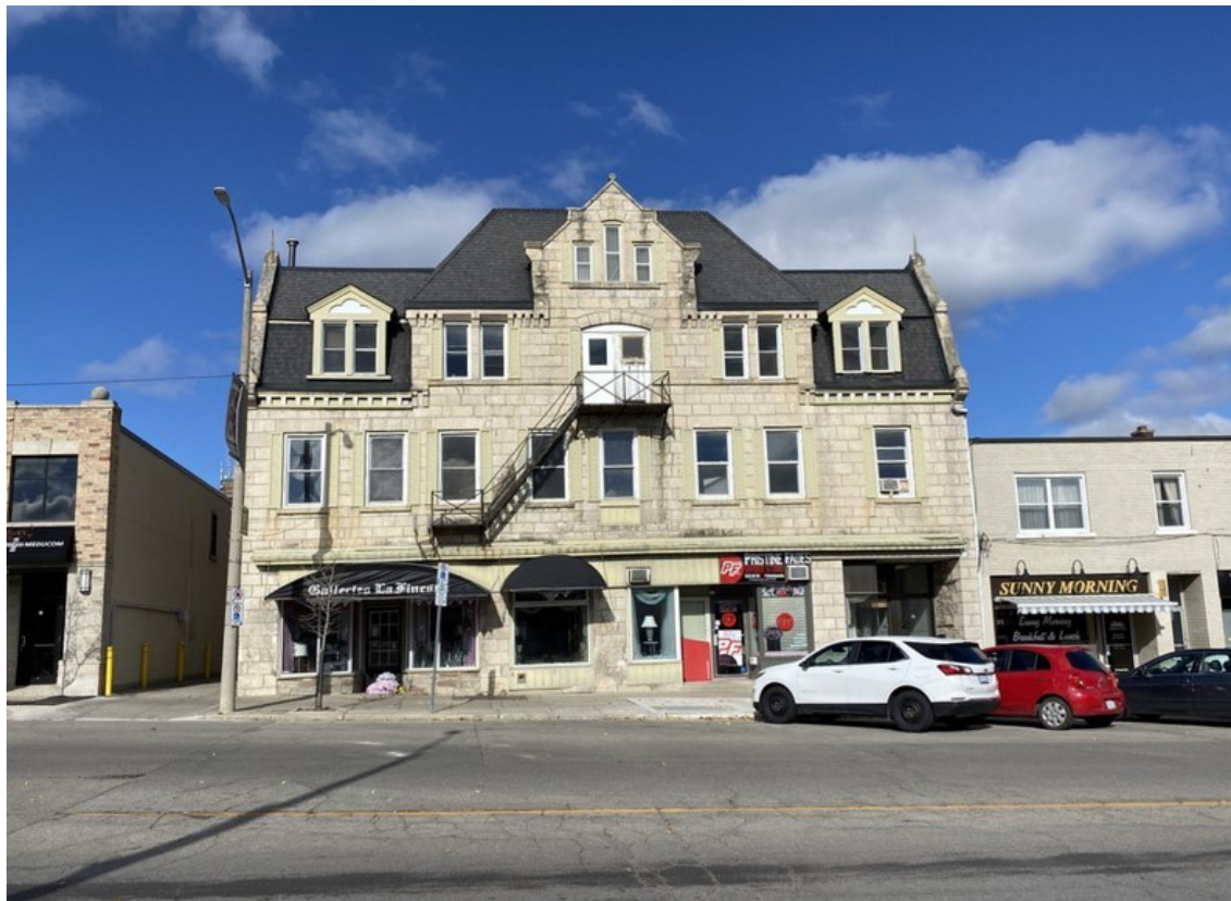
Figure 20: The former Union Hotel on Macdonell Street, constructed of local limestone (A.S.I., 2023).
