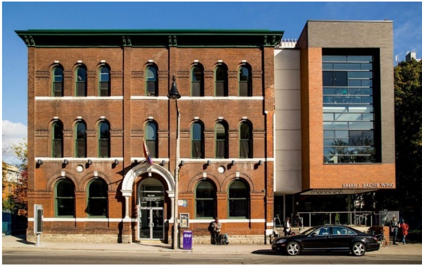
Figure 34: Example of addition to heritage building using visually and physically consistent material (brick) on the primary structure of the exterior wall, and contemporary material (concrete) on the secondary structure of the exterior wall. Address: 519 Church Street, Toronto (Vik Pahwa, 2014).
