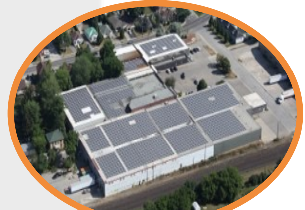
Moose Power Alum: 460 Industrial, Woodstock (Brookfield) Built in 2011, one of the largest rooftop solar projects in Ontario at the time
