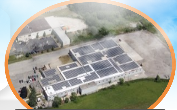
Moose Power Alum: 80 Norwich, Woodstock (Brookfield) Built in 2011, one of the largest rooftop solar projects in Ontario at the time
