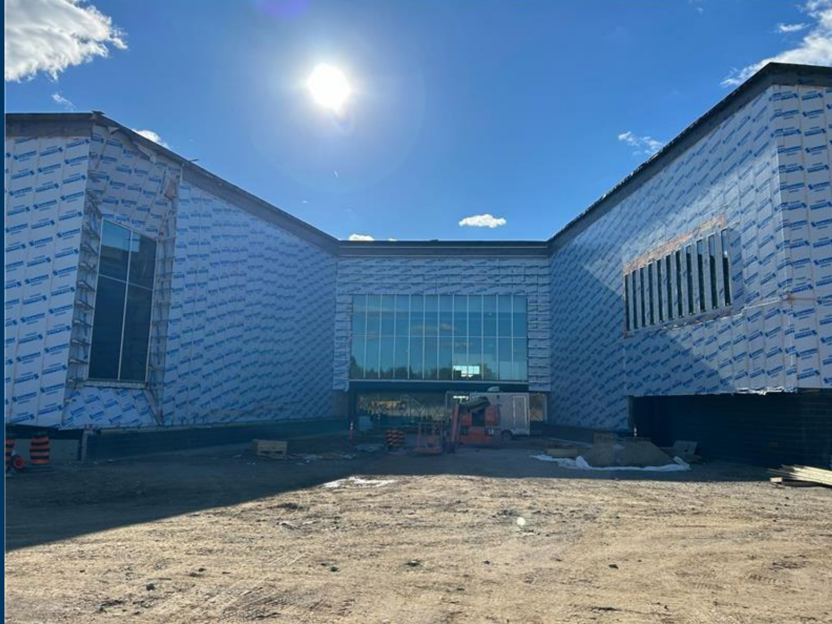
📍 South End Community Centre under construction
