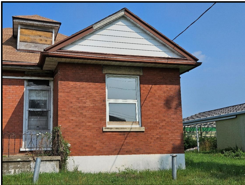
Image 2: 316 Grange Road – Residence Façade Projecting Bay (Photo taken July 22, 2025; Facing Northwest)
