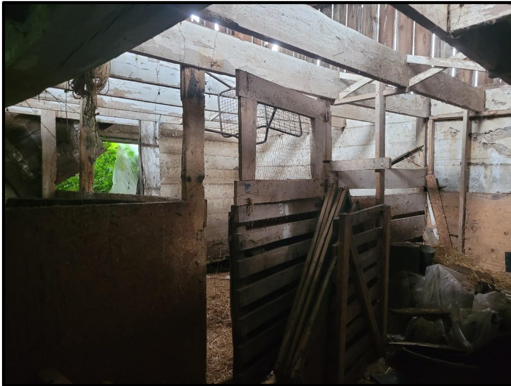
Image 43: Timber Frame Barn – First Floor Interior (Photo taken August 15, 2023)
