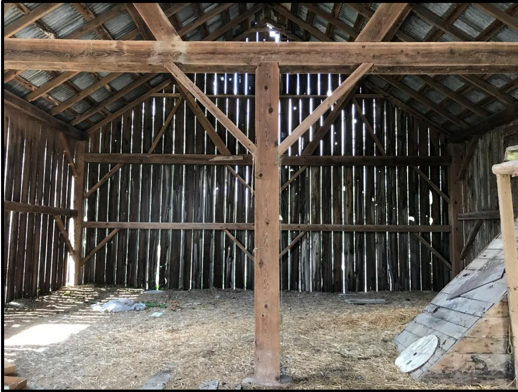
Image 39: 316 Grange Road – Interior of Timber Barn (Photo taken July 14, 2021)
