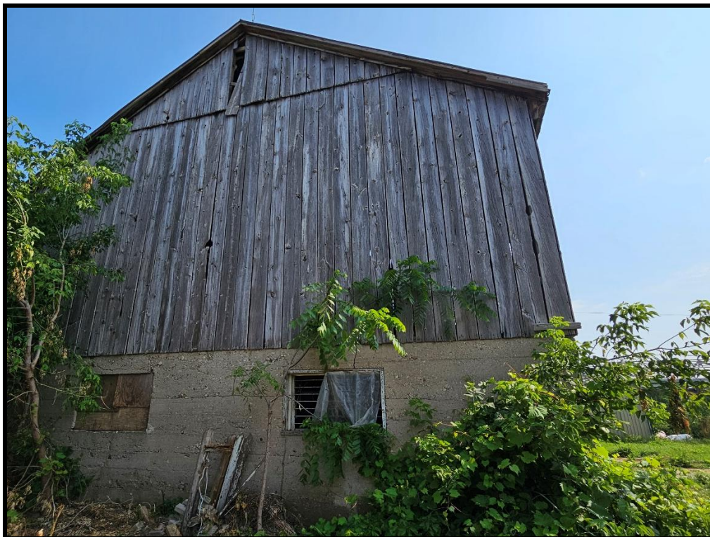
Image 16: 316 Grange Road – Timber Barn Southwest Elevation (Photo taken July 22, 2025; Facing Northeast)
