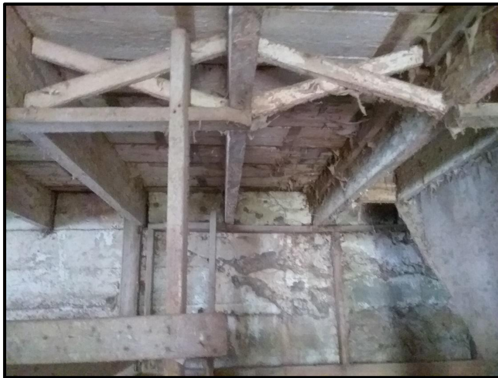
Image 44: Cross Bridging Visible on Upper Floor Joists (Photo taken July 7, 2021)
