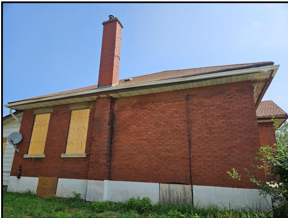
Image 4: 316 Grange Road – Residence Southwest Elevation (Photo taken July 22, 2025; Facing Northeast)
