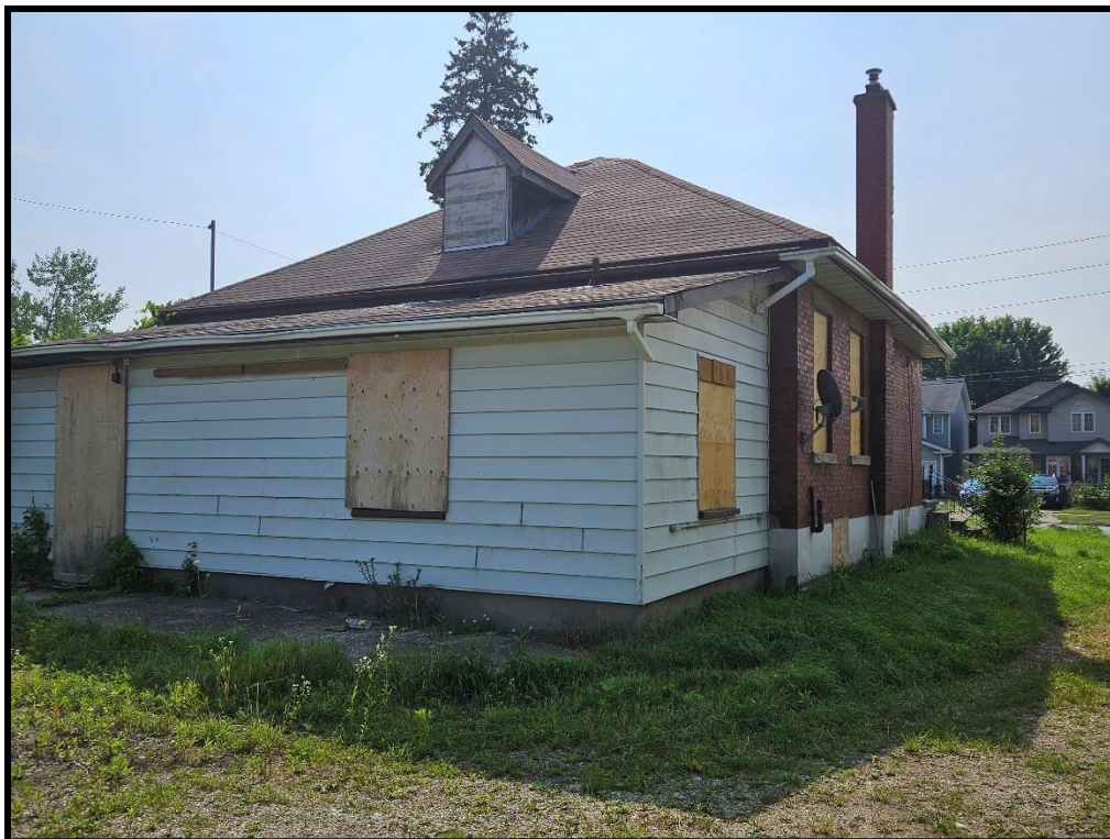
Image 6: 316 Grange Road – Residence West Corner View (Photo taken July 22, 2025; Facing East)
