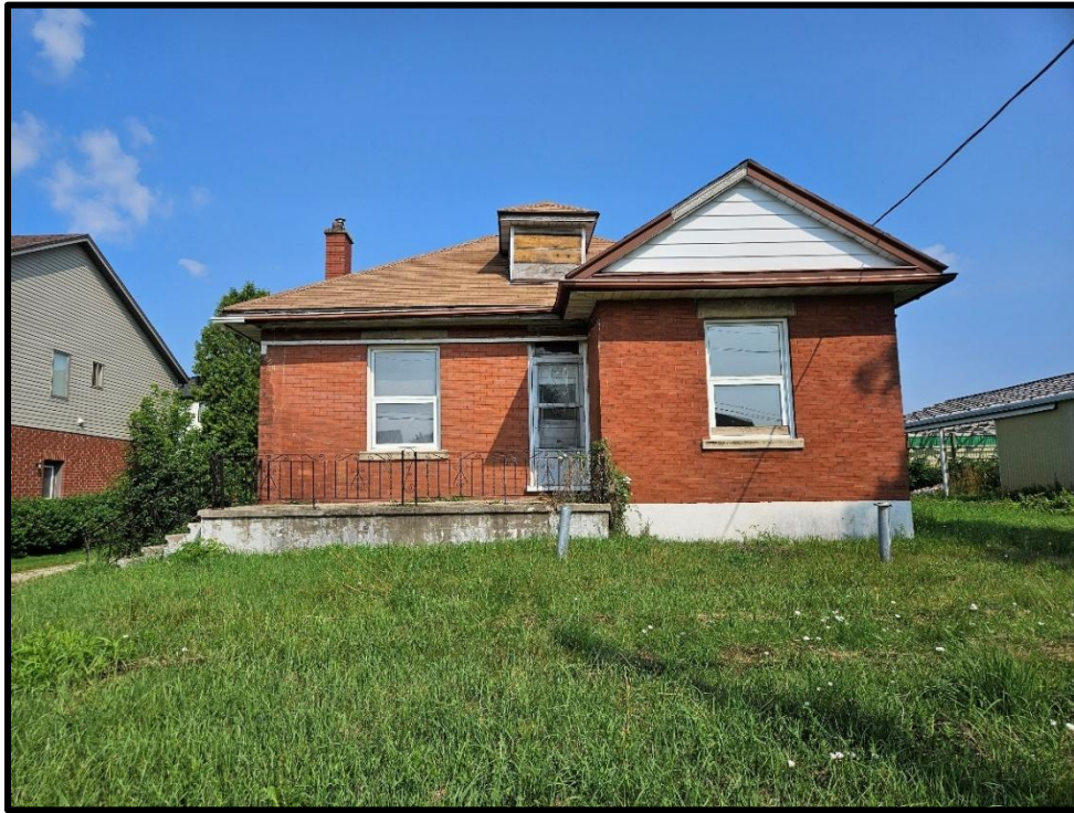
Image 1: 316 Grange Road – Residence Façade (Southeast Elevation) (Photo taken July 22, 2025; Facing Northwest)
