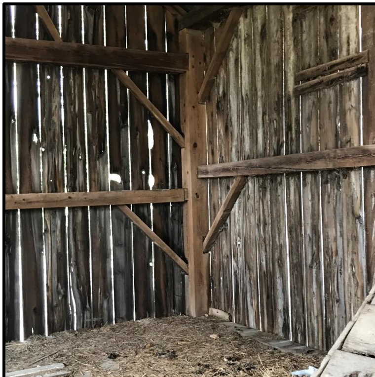
Image 40: 316 Grange Road – Interior of Timber Barn (Photo taken July 14, 2021)
