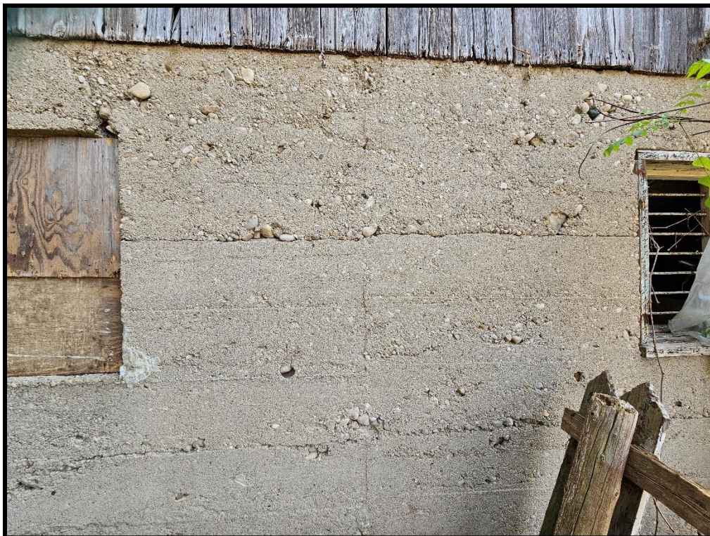
Image 18: 316 Grange Road – Detail of Timber Barn Concrete Foundation (Photo taken July 22, 2025; Facing Northeast)
