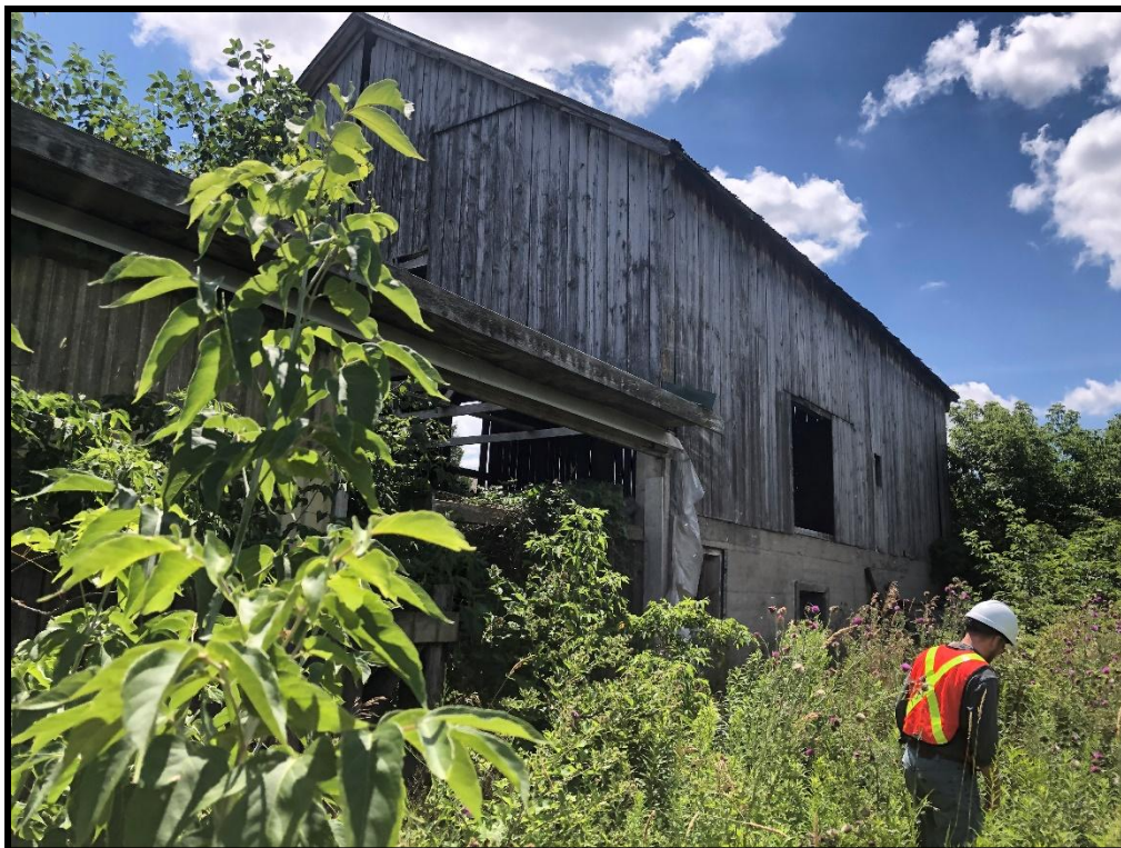
Image 20: 316 Grange Road – Timber Barn Northwest Elevation (Photo taken July 22, 2025; Facing Southwest)
