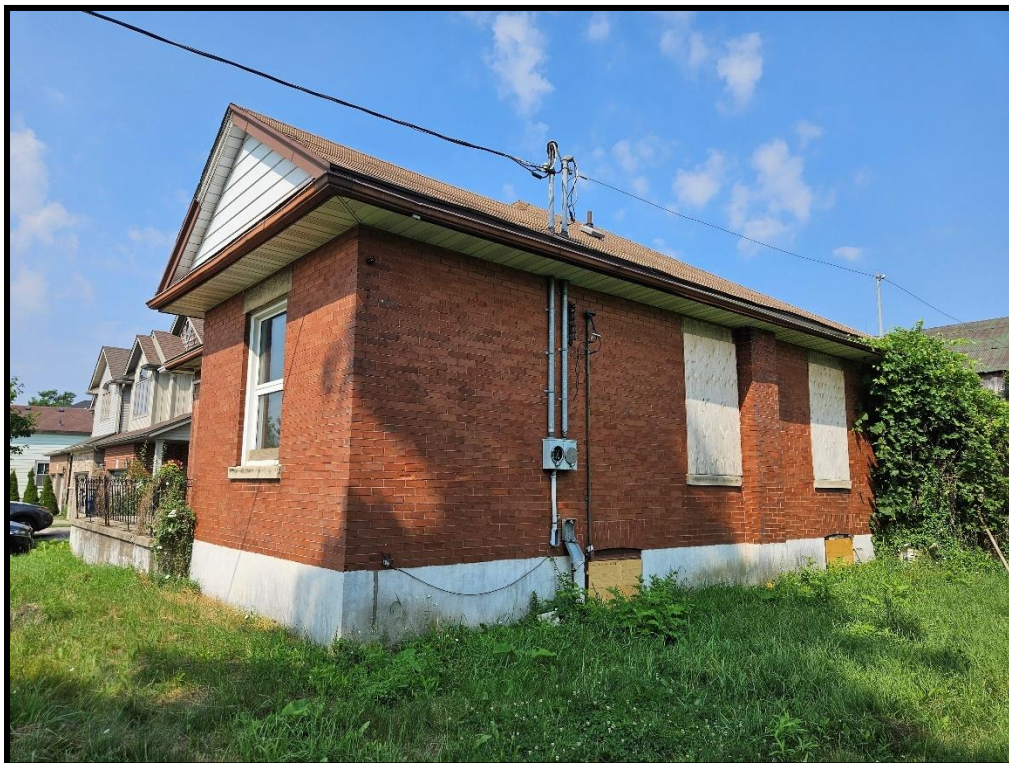
Image 10: 316 Grange Road – Residence Northeast Elevation (Photo taken July 22, 2025; Facing Southwest)
