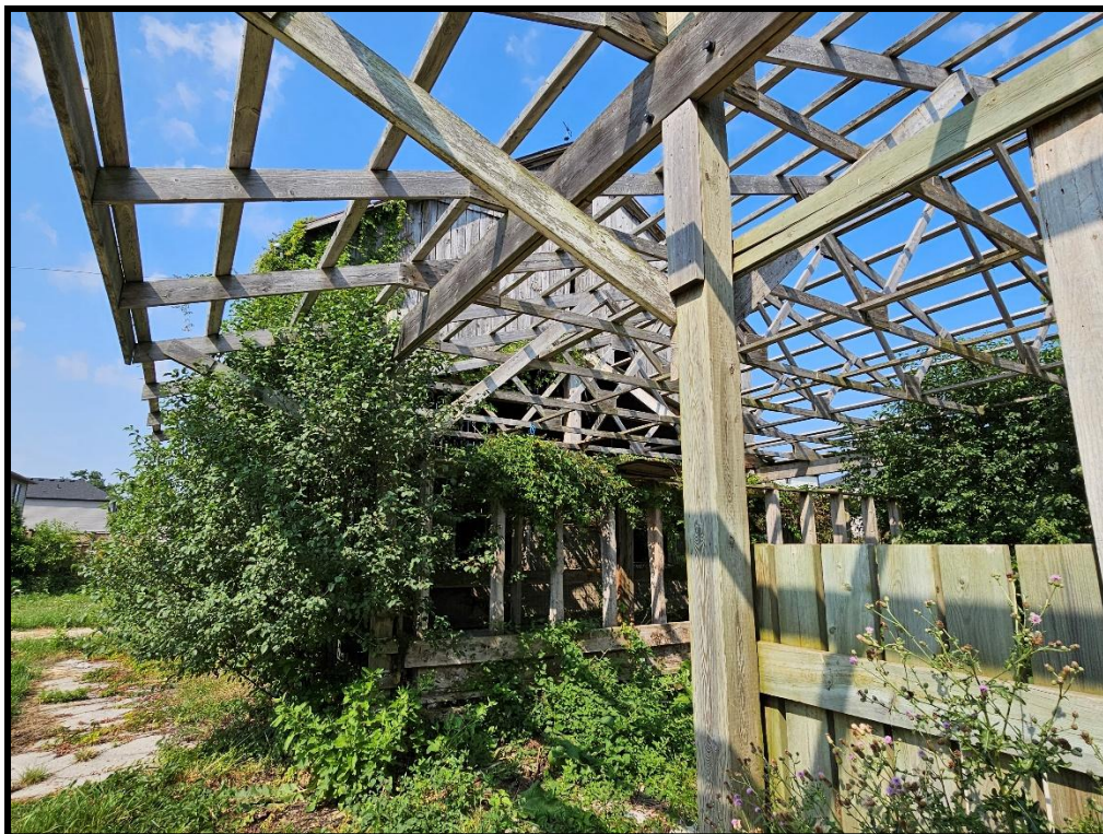
Image 26: 316 Grange Road – Timber Barn Wood Frame Addition (Photo taken July 22, 2025; Facing West)
