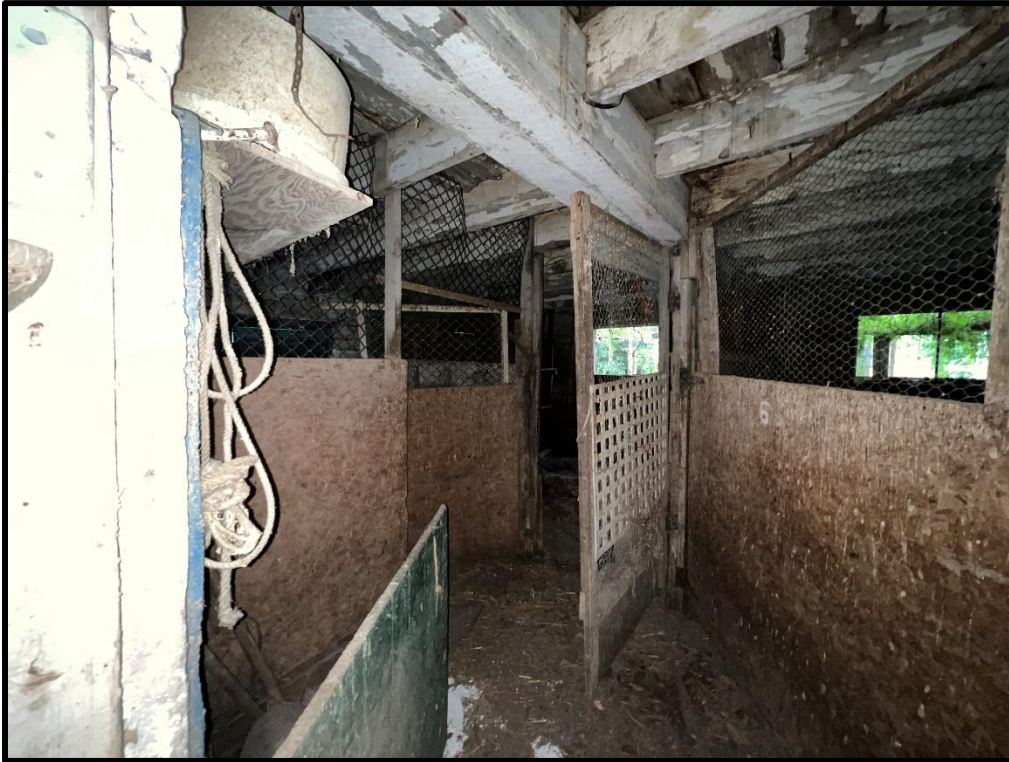
Image 45: Timber Frame Barn – First Floor Interior (Photo taken August 15, 2023)
