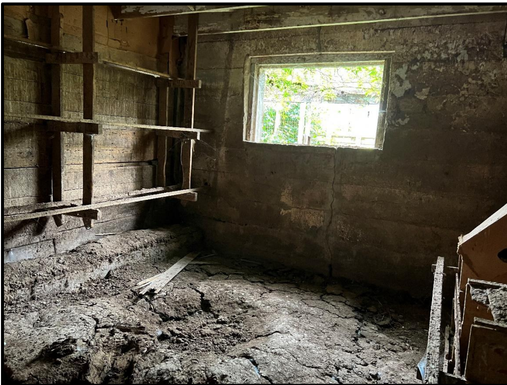
Image 46: Timber Frame Barn – First Floor Interior (Photo taken August 15, 2023)
