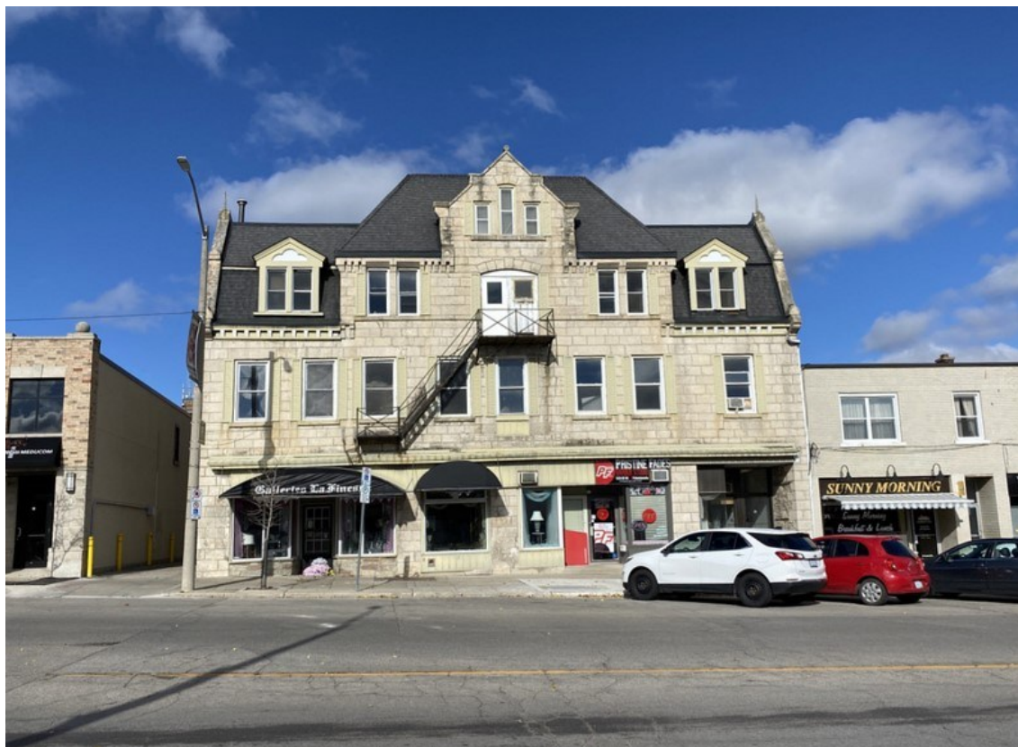
Figure 20: The former Union Hotel on Macdonell Street, constructed of local limestone (A.S.I., 2023).
