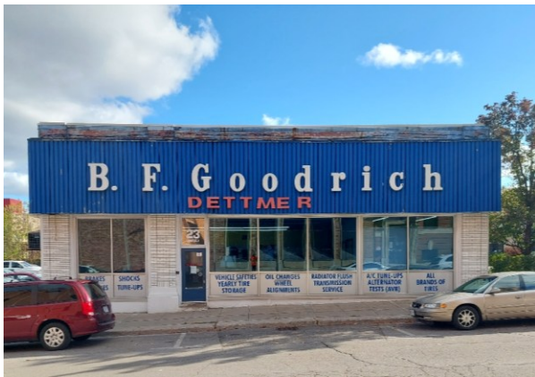
Figure 29: Dettmer Tire building with current cladding (A.S.I. 2023).
