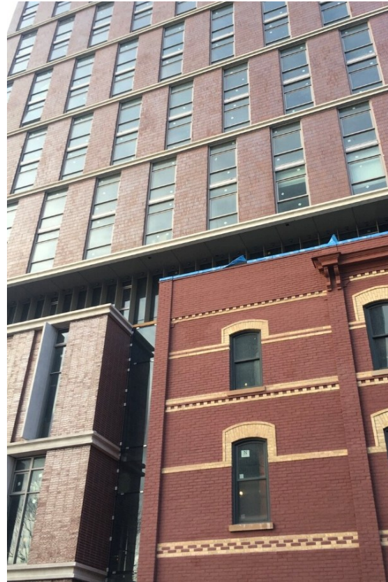
Figure 39: Detail of 700 Spadina Avenue, Toronto illustrating compatible materials (existing and new brick) separated by a physically articulated gap in a distinct material (glass) (Urban Toronto Database).
