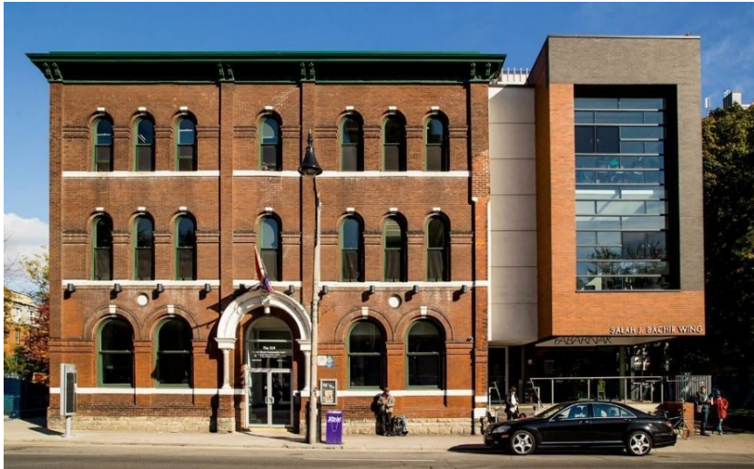
Figure 37: Example of addition to heritage building using visually and physically consistent material (stone) on the primary structure of the exterior wall, and contemporary cladding (glass) on the secondary structure of the exterior wall. Address: 144 Wellington Street, Ottawa (Doublespace Photography, 2015).
