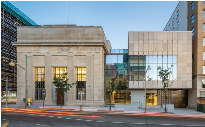
Figure 37: Example of addition to heritage building using visually and physically consistent material (stone) on the primary structure of the exterior wall, and contemporary cladding (glass) on the secondary structure of the exterior wall. Address: 144 Wellington Street, Ottawa (Doublespace Photography, 2015).
