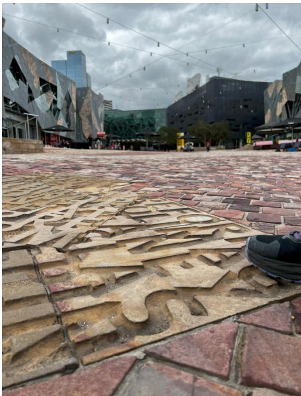
Figure 52: Although this paving treatment helps to identify the public Fed Square in Melbourne, Australia, the rough surface would not be compliant with accessibility standards in the City of Guelph (Mark Steele, 2023).
